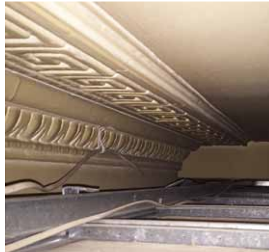
Fig. A25 Original cornice rear room ground floor (above modern suspended ceiling)
