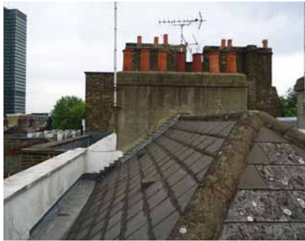
Fig. A48 Main roof
