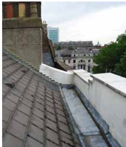
Fig. A51 Main roof
