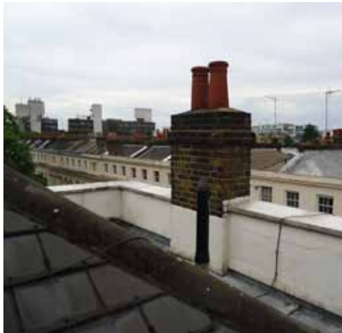
Fig. A50 Main roof
