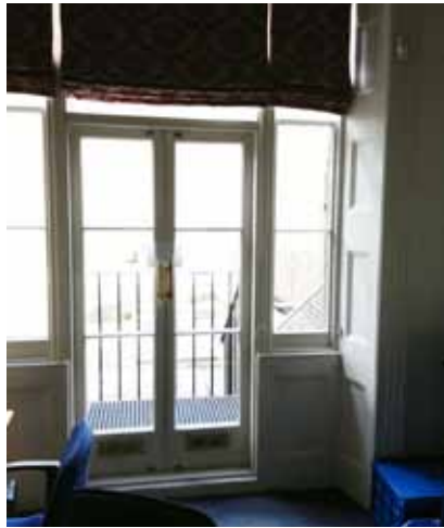
Fig. A33 1st floor - rear office
