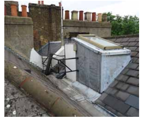
Fig. A49 Main roof
