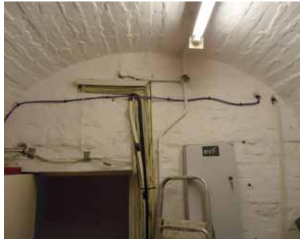
Fig. A11 Lower ground floor - wine vault
