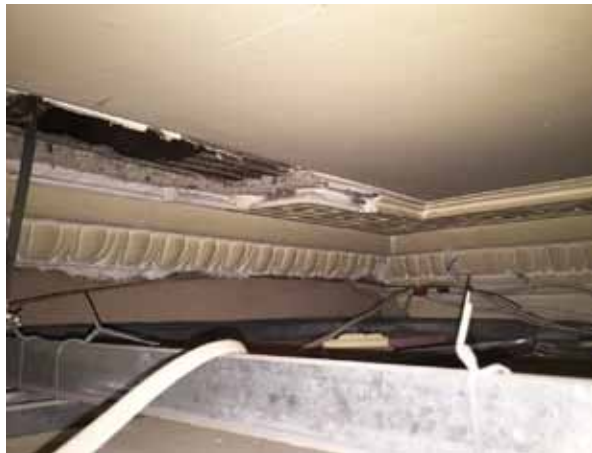
Fig. A36 Original cornice rear room first floor (above modern suspended ceiling)
