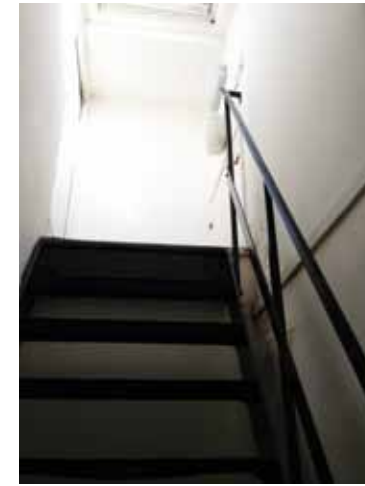
Fig. A44 3rd floor - stairs to roof
