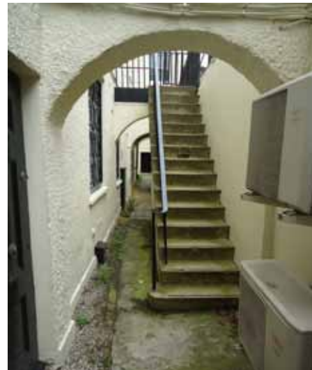
Fig. A9 Side lightwell - steps to street
