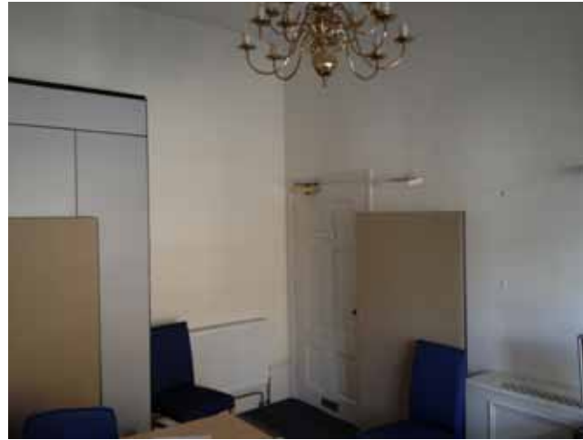
Fig. A34 1st floor - rear office
