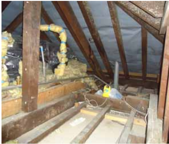
Fig. A47 Loft space front roof
