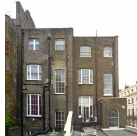
Fig. A4 View of rear elevation
