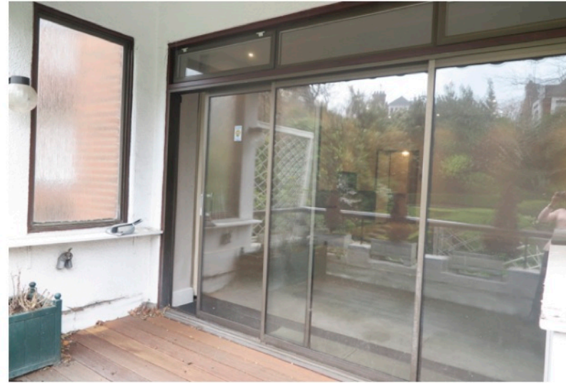
First Floor Balcony 02
