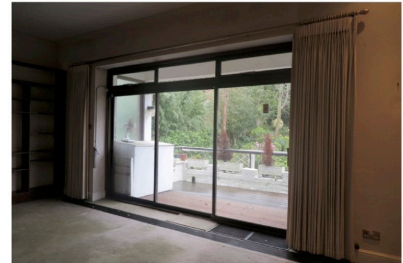
First Floor Balcony 03
