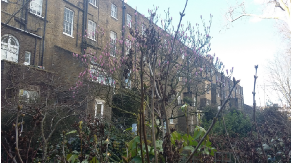
View of rear of wider terrace (looking North)
