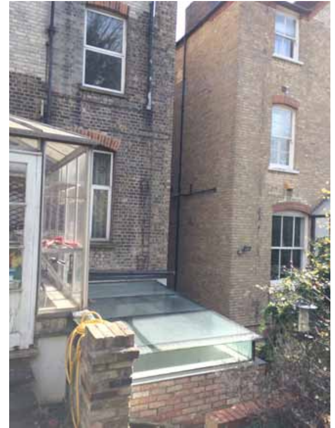
Rear view of no. 40 Arkwright Road, showing existing glass roof over lower ground floor extension
