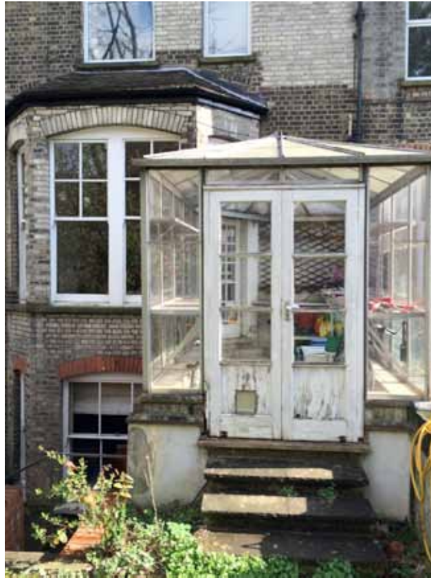
Rear view of no. 40 Arkwright Road, showing existing dilapidated conservatory, rebuilt part of rear wall, and unsympathetic uPVC windows at first floor level
