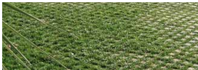
Example of green parking system
