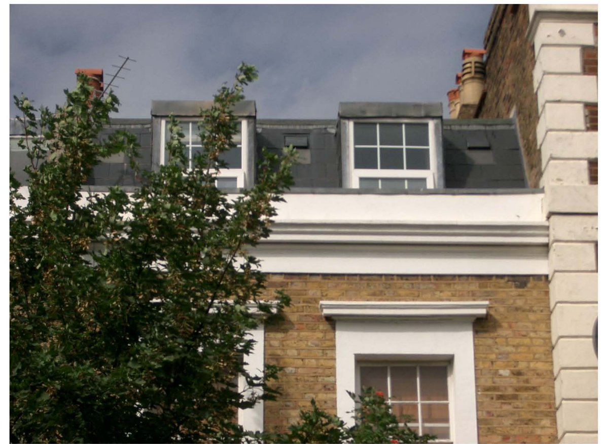
Front View at Existing Loft Conversions at 183 Leighton Road (as proposed for Number 175)
