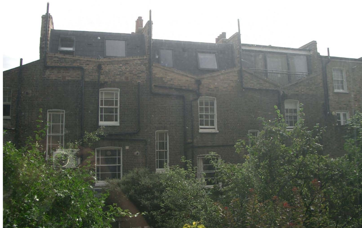
Rear View at Existing Loft Conversions at 165 - 161 Leighton Road
