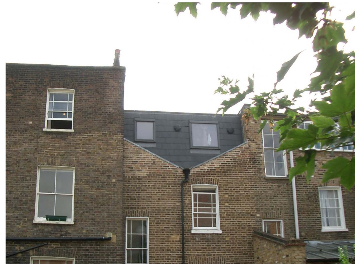
Rear View at Existing Loft Conversions at 183 - 179 Leighton Road
