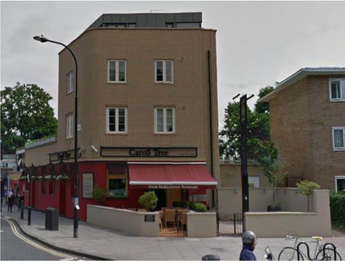
Figure 7 (above): Front elevation of appeal site from Highgate Road in June 2014 (Source: Google Streetview). Note: forecourt has now been divided into two.
