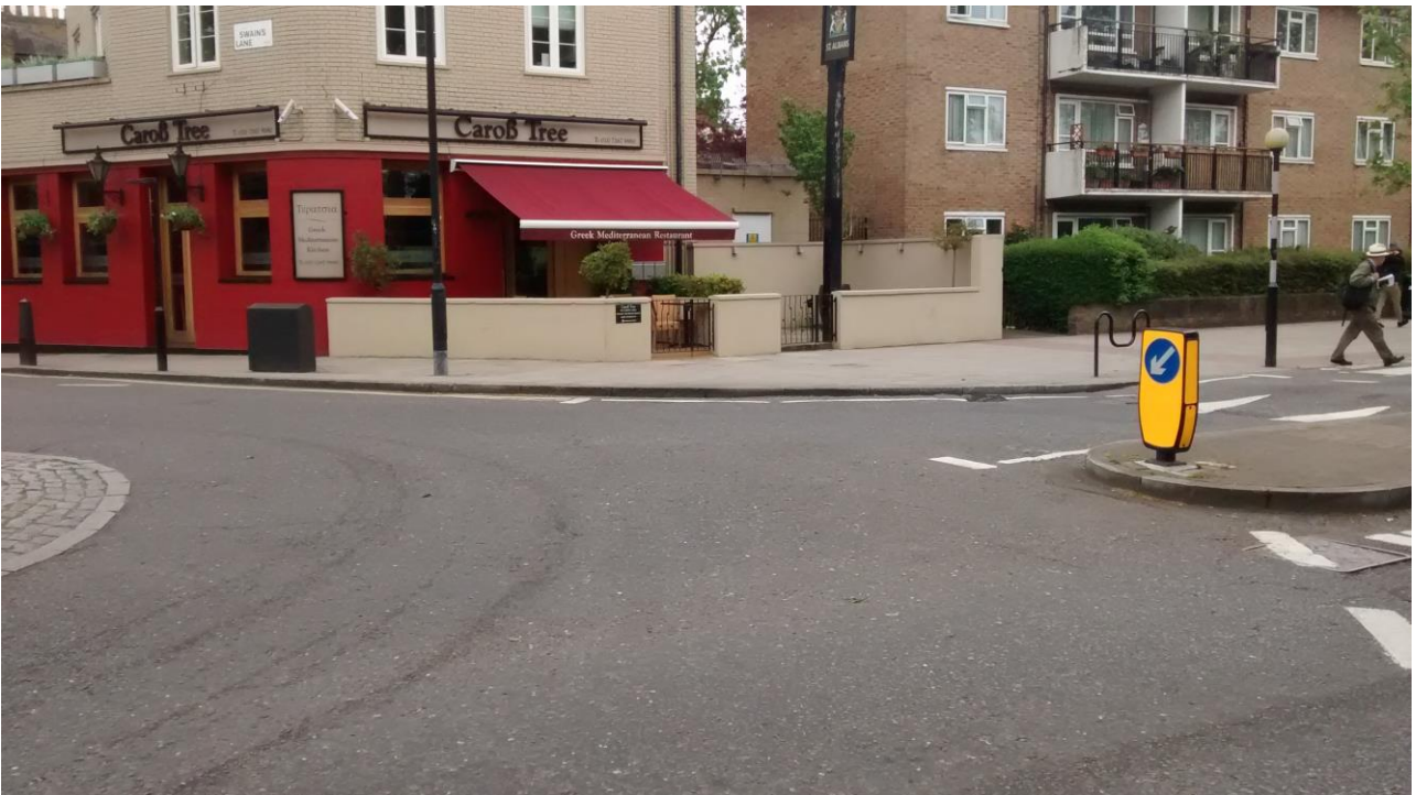
Figure 8 (above): Front/side elevation of appeal site from junction of Swain's Lane and Highgate Road in May 2016
