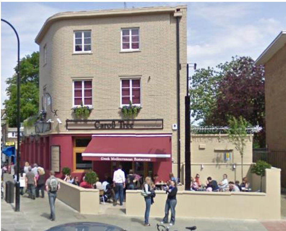
Figure 6 (above): Front elevation of appeal site from Highgate Road in May 2009 (Source: Google Streetview). Note: mature tree removed, boundary treatment altered.
