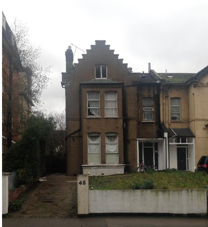
Photo 1: The existing site
