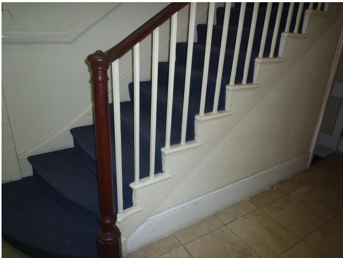
Fig.15 The main stair
