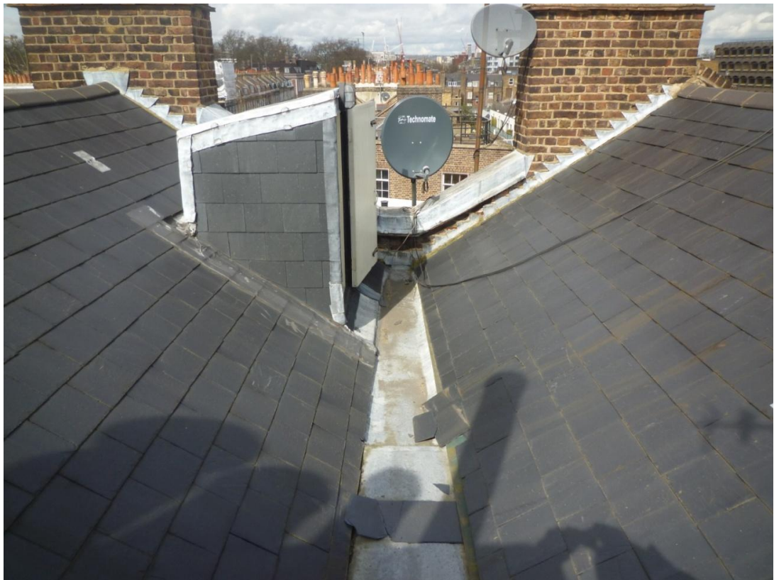
Fig. 19 The valley between the two roof ridges
