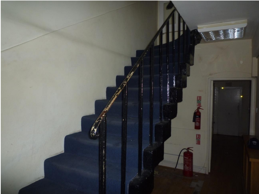
Fig.12 Stair from basement to ground floor
