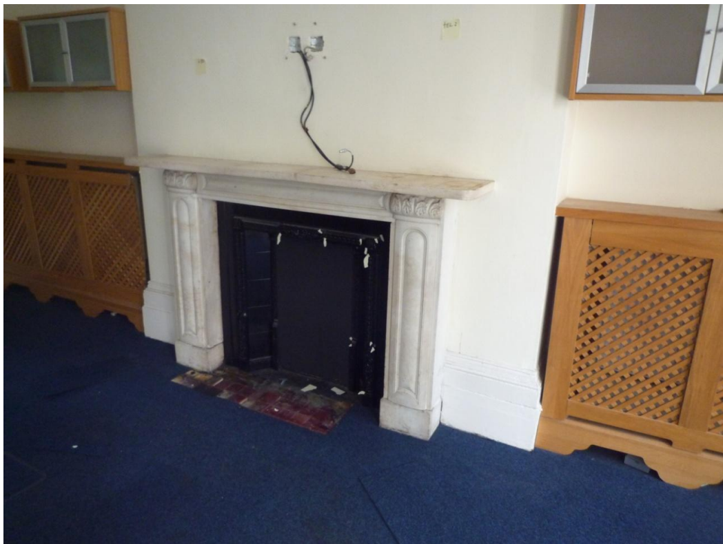
Fig.17 Chimney piece in the first floor front room
