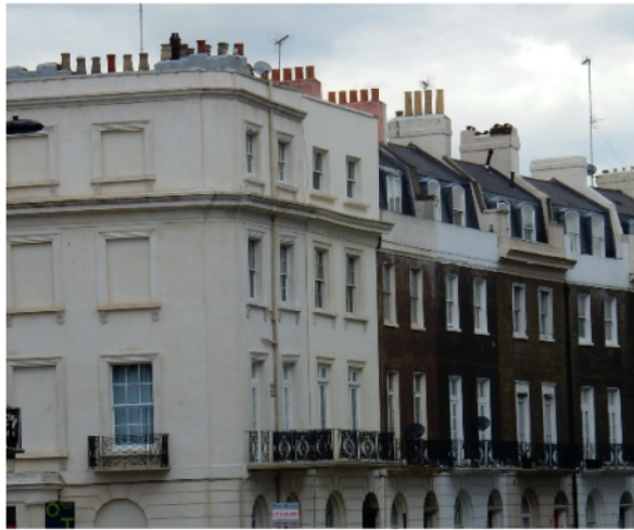
Fig 9. Corner of Mornington Place (No. 25)
