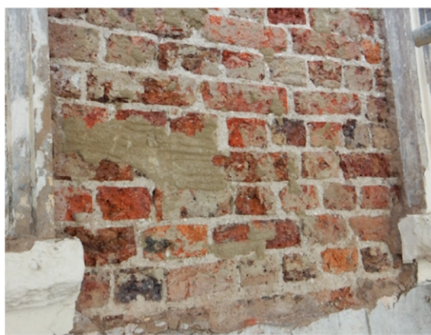
Fig.8 Wall at mid height in fair condition.
