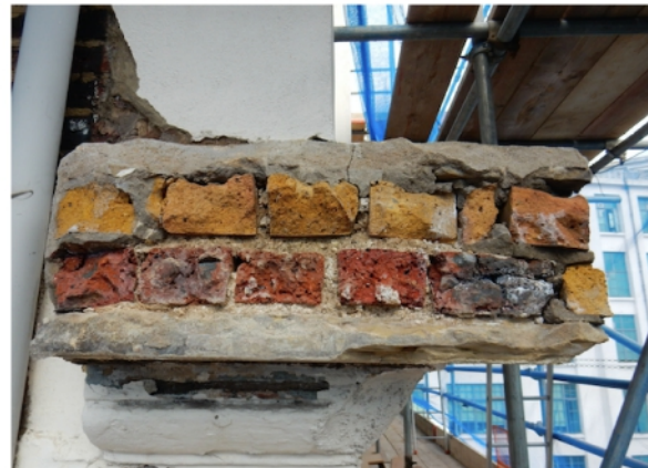
Fig.12 South cornice (west end)
