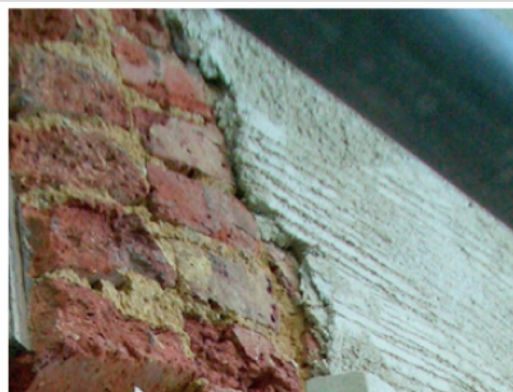
First coat up to 10mm thick
