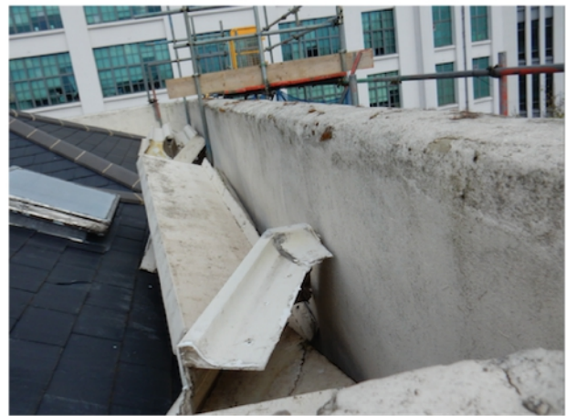
Fig. 2 Rear of south parapet
