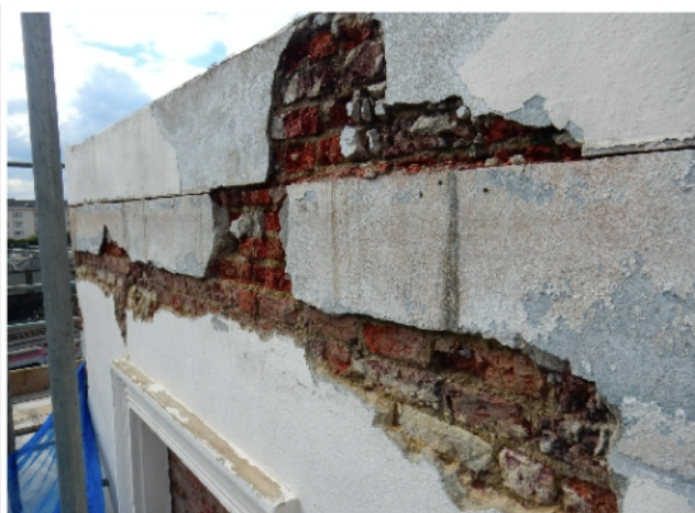
Fig. 5 Parapet on south side
