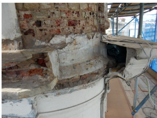
Fig. 7. Detail of mid height cornice
