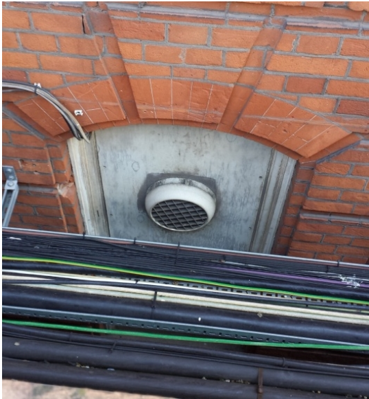
(image 3) Existing Window view from Queen Square at ground level, looking across lightwell, down to basement level, at one of the affected windows.
