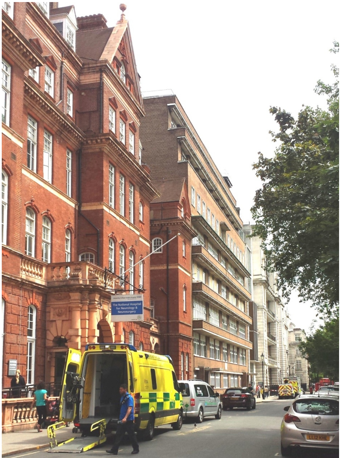
(image 1) Existing Building
