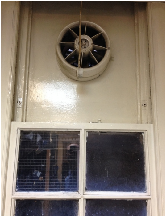
(image 4) Existing Window Internal view
