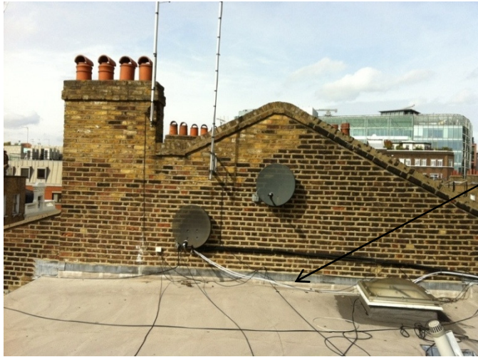
104 Cleveland Street roof looking north
