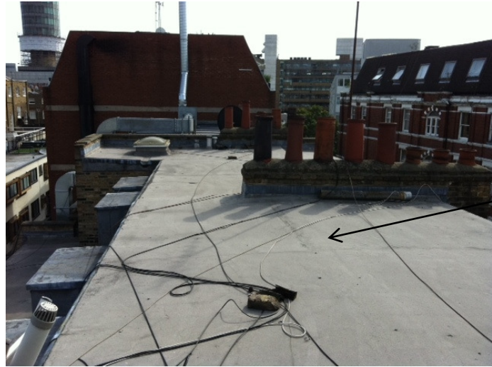
104 Cleveland Street roof looking south
