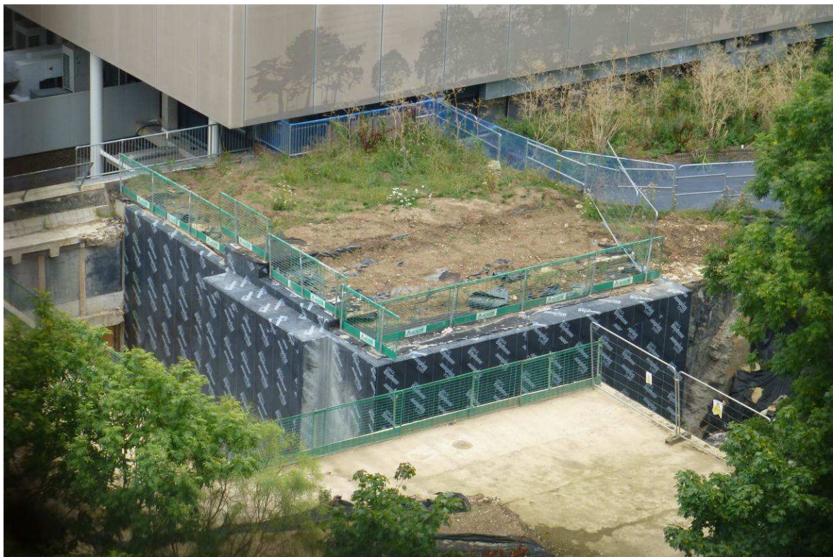
Photo 13. View from St Stephens Tower of north end of linear accelerator.
