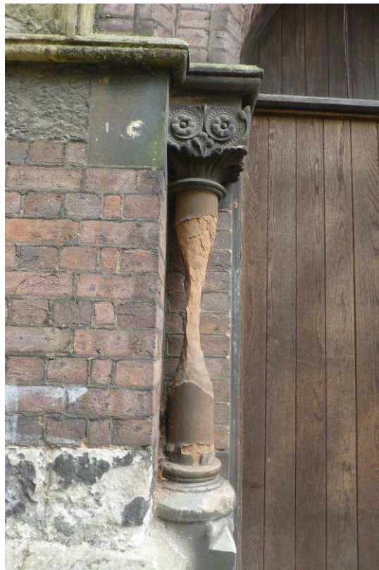
Photo 5. Sandstone decorative column to north porch.
