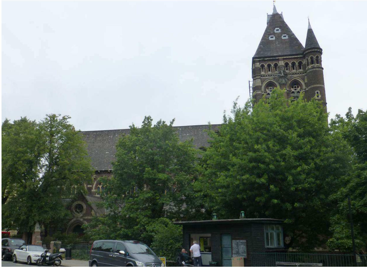
Photo 1. St Stephens South elevation
