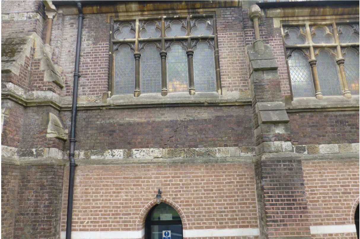
Photo 2. Distortion to the east end of the north aisle externally
