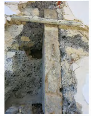
350mm deep beamx300 wide formed with double web.
