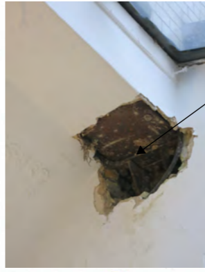
160 square column supporting 355mm wide double webbed beam
