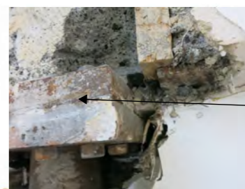
160 diameter circular column, with 320x360x60thk capping plate
