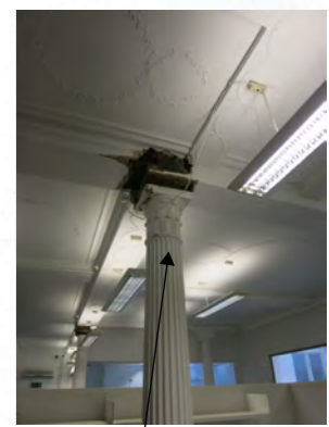
350mm deep beamx300 wide formed with double web.
