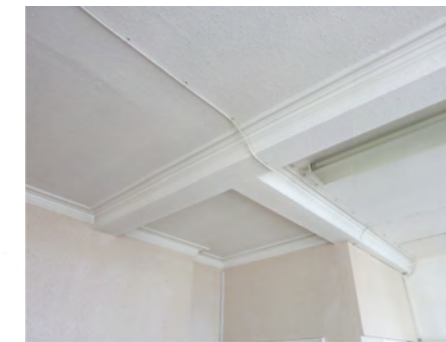
Encased downstand beams
