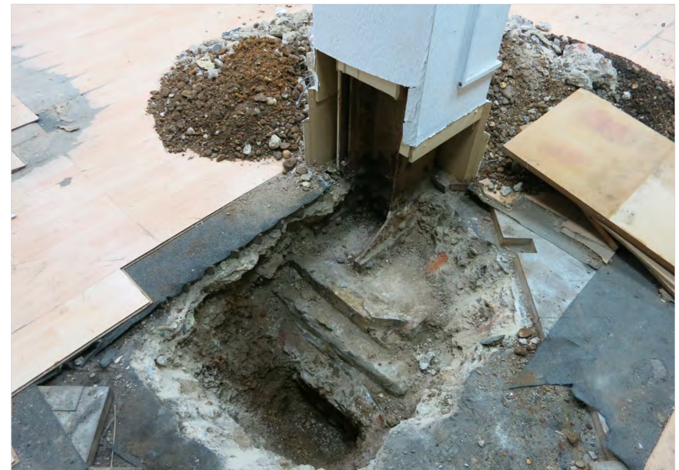
Existing pad footings under columns
