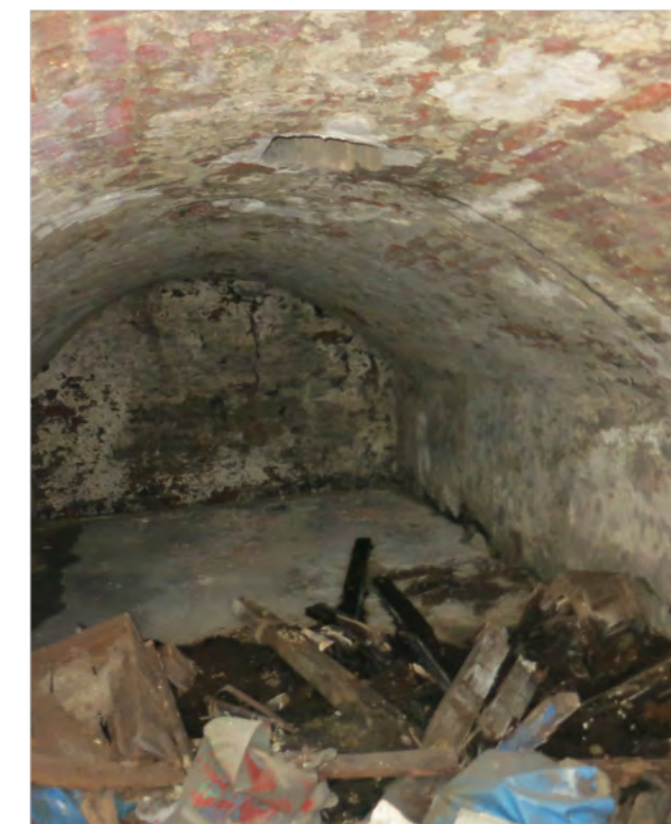
View of existing vault structure
