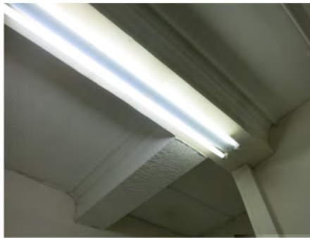
Original ceiling and downstand visible
