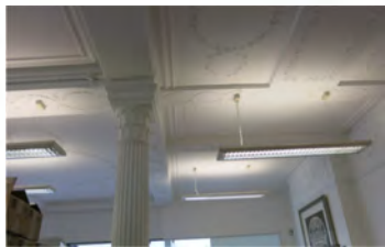
Architecturally encased column
