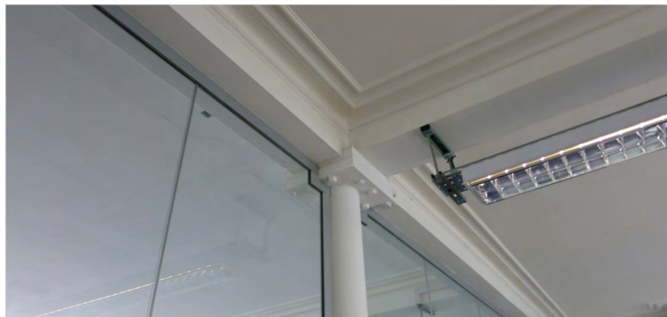
Existing beam and column junction
