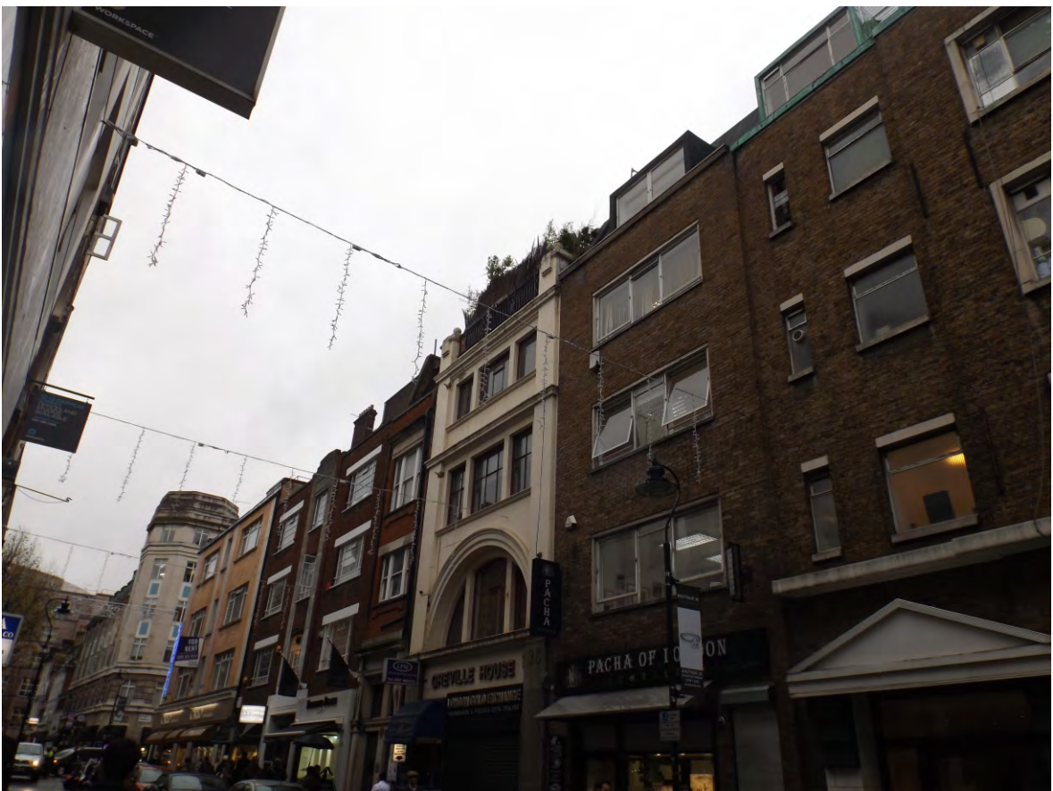
Appendix 2.4: Views from Greville Street showing enclosed nature
