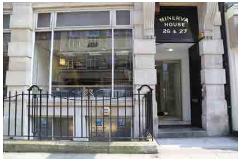
2_ 11.03.216 - Hatton Garden - existing entrance
