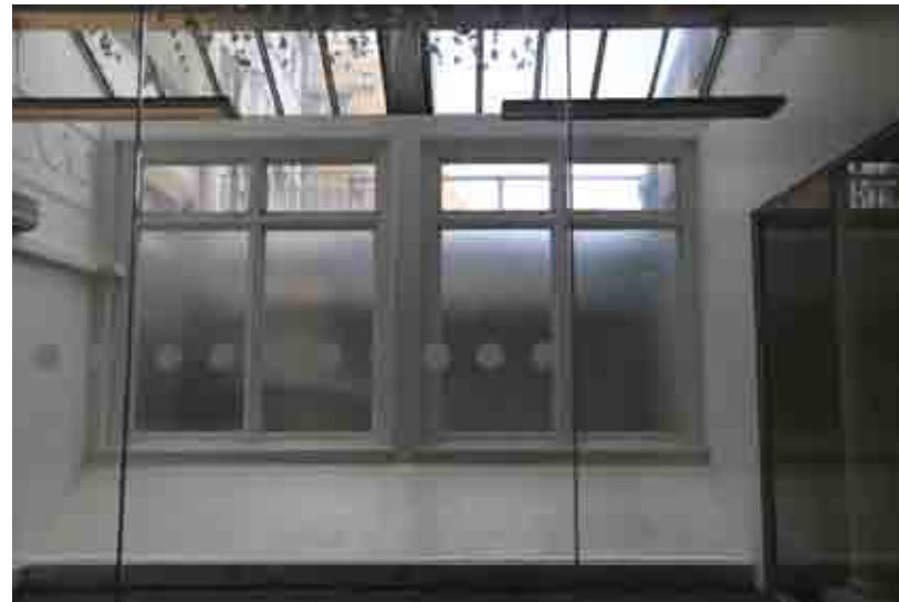
2_ 11.03.216 - View from the ground floor looking the glass-roof
