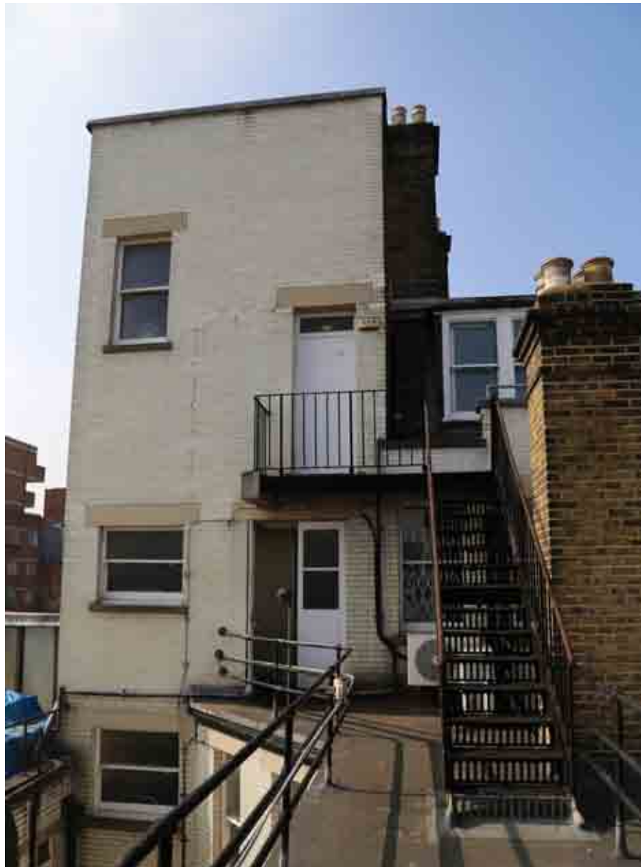
1_ 11.03.2016 - View from the third floor roof looking the front building
