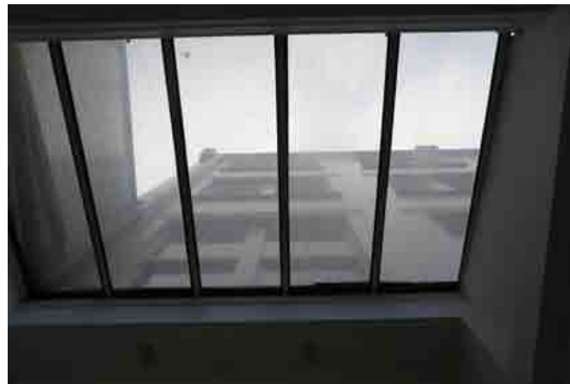
3_ 11.03.216 - View from the ground floor looking the glass-roof
