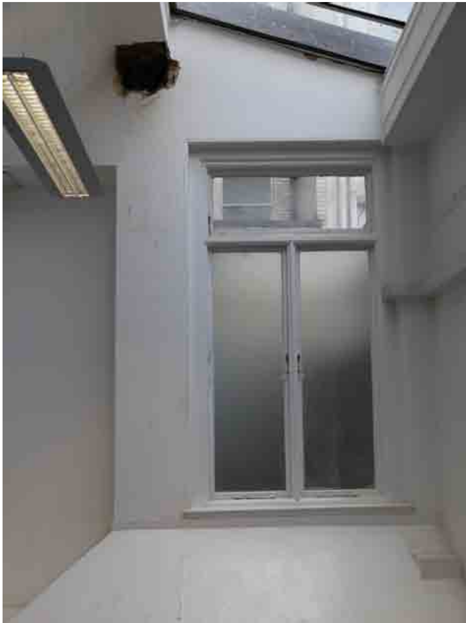
1_ 02.06.215 - View from ground floor to the lightwell
