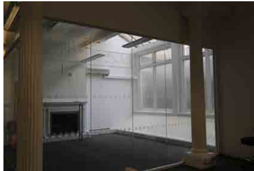
3_ 11.03.216 - View from the ground floor to the existing glassroof
