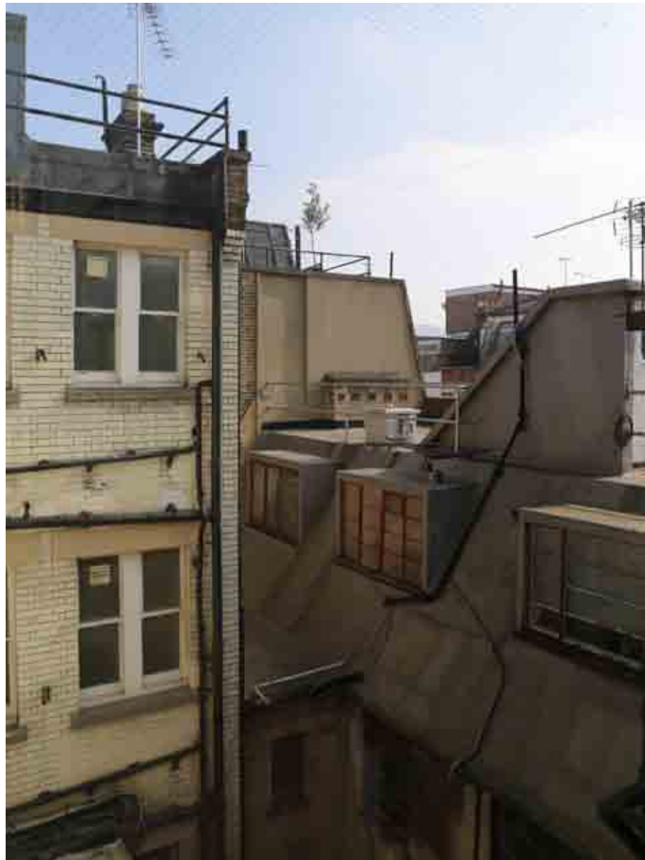
1_ 11.03.2016 - View from the third floor looking the lightwell
