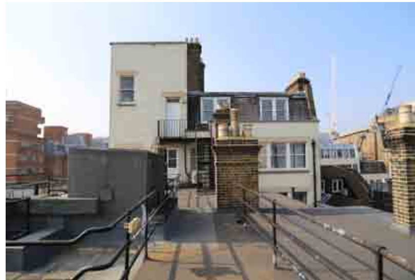
2_ 11.03.216 - View from the third floor roof looking the front building
