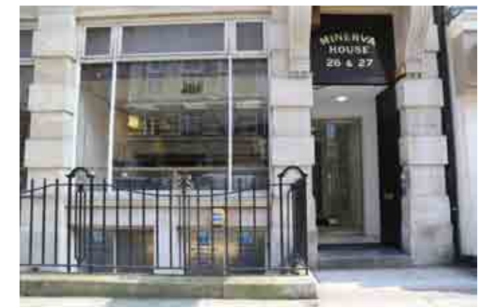
Hatton Garden - existing entrance
