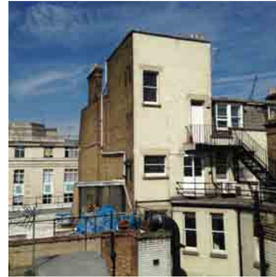
Existing South Courtyard - view from roof
