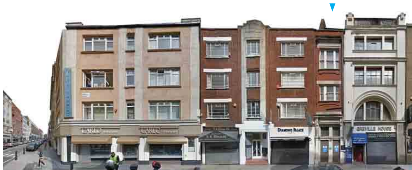
View along Greville Street from the South-East
