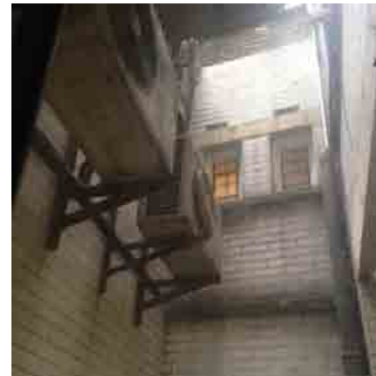
Existing South Courtyard - view from basement
