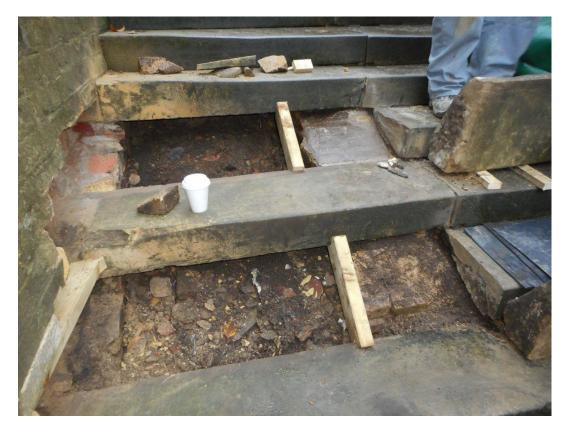
Image taken during opening up works showing the treads have an inclined soffit bearing on a strip foundation support of unknown depth and quality. Treads are built into the side walls.
