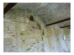
• There is serious cracking at the central arch opening carrying the vault over the steps.
