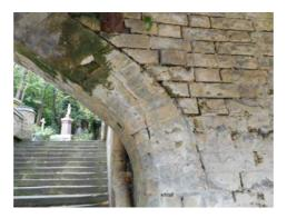
• The flanking walls to the steps have a large crack roughly where the vault structures behind them end and they become retaining walls
