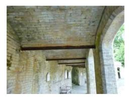
• The rear wall of the loggia (which has burial vaults behind it) suffers from extensive water penetration, largely from the top. It has been repointed in patches in the past with an unsuitable cement-rich pointing, and has extensive areas where the pointing has failed completely. The pointing that remains is contributing to problems and is unsightly. There are numerous failed or broken bricks, some associated with the fixing of memorial plaques which have now disappeared.
