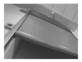
Components can be powder coated. It may be possible to conceal both head box and guide rails by plasterboard cladding, they will additionally project into the room geometry.
