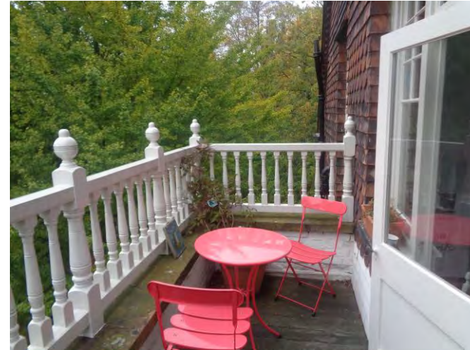
Figure 11: New timber balustrade that matches the original to no.7.
