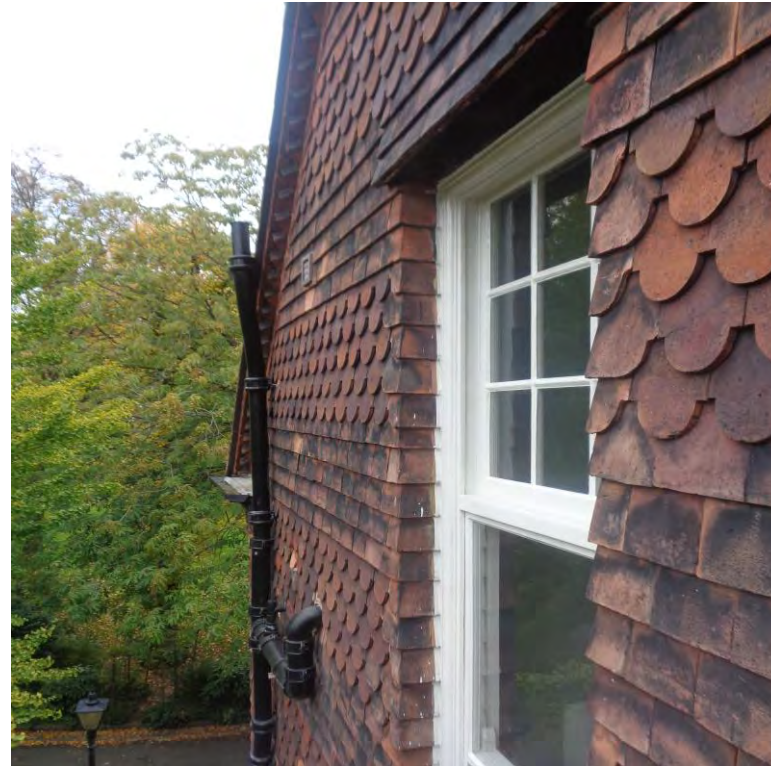
Figure 22: Tile hanging on the side elevation.
