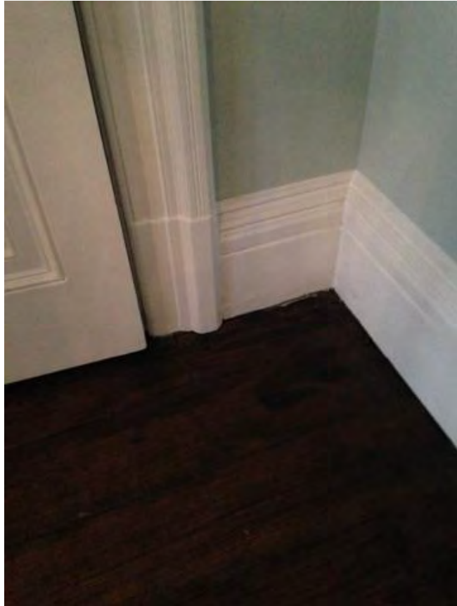
Figure 25: Doors, skirting and architraves in the rear room at ground floor level.
