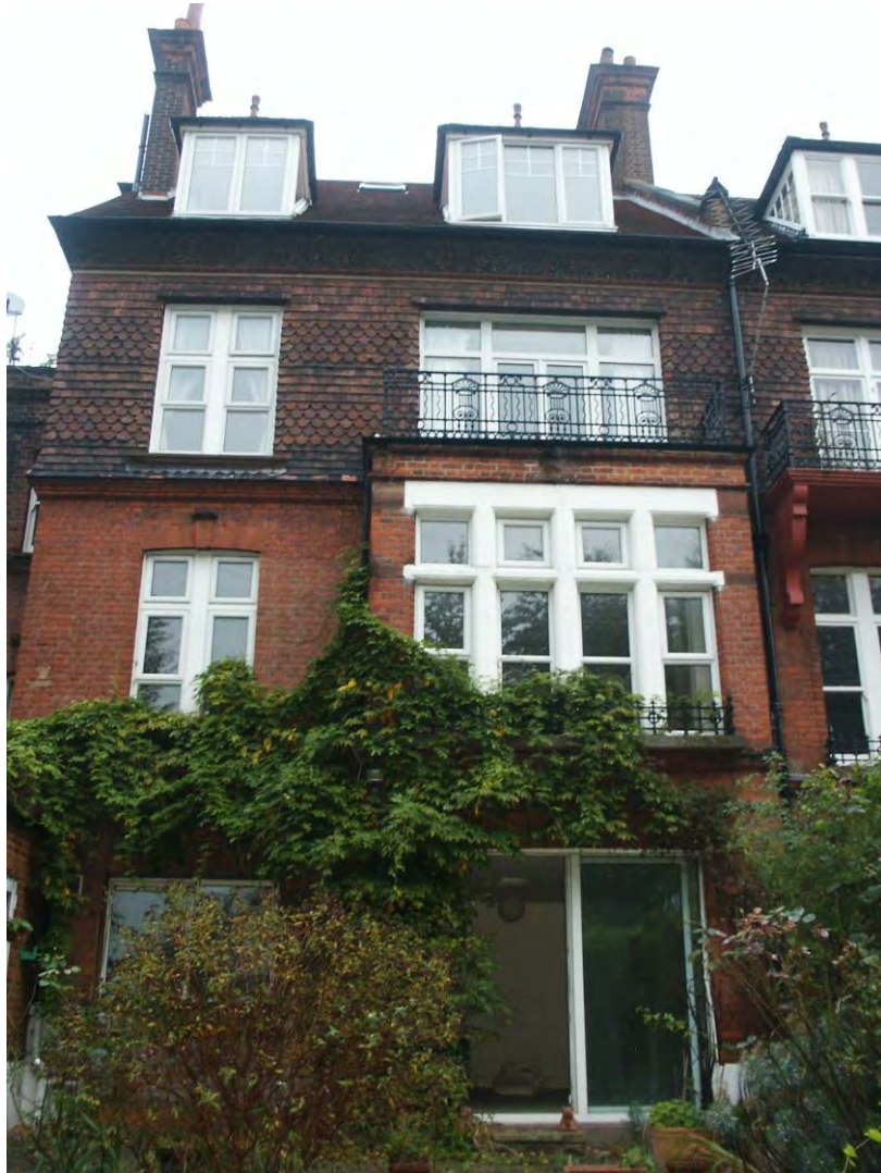
Figure 20: Rear elevation prior to works to replace UPVC windows
