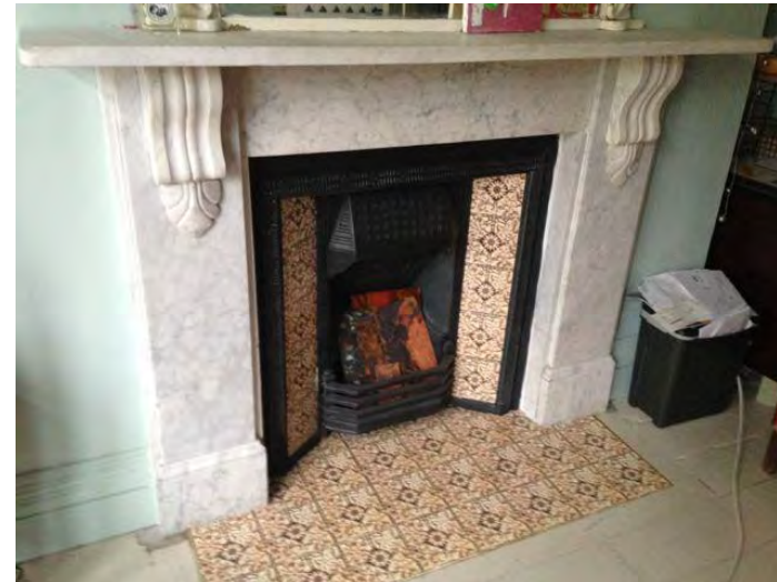
Figure 12: Reinstated fireplace and tiles in front room at first floor level.
