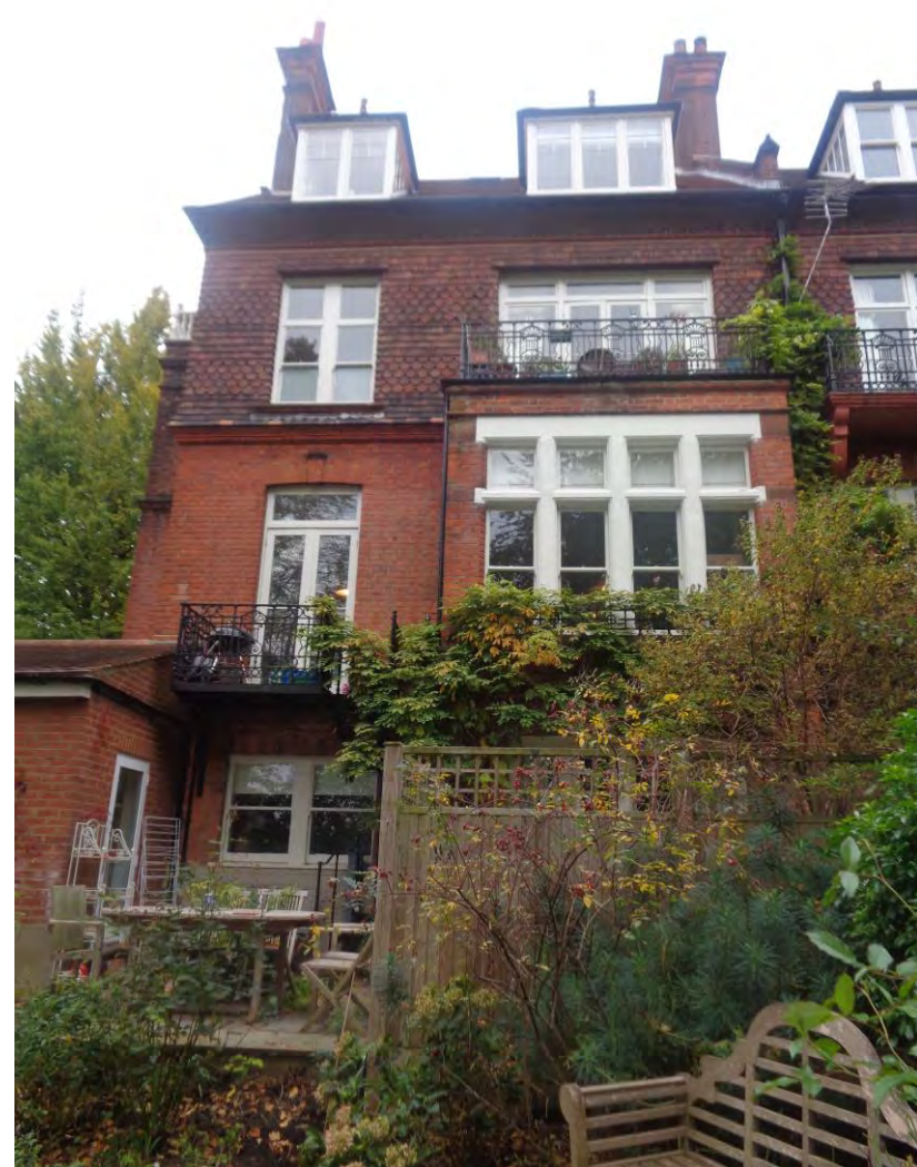
Figure 21: Rear elevation in its current state. UPVC windows were replaced with timber casements; to match those on the other buildings in the group. Window behind timber fence was also replaced with timber French windows.
