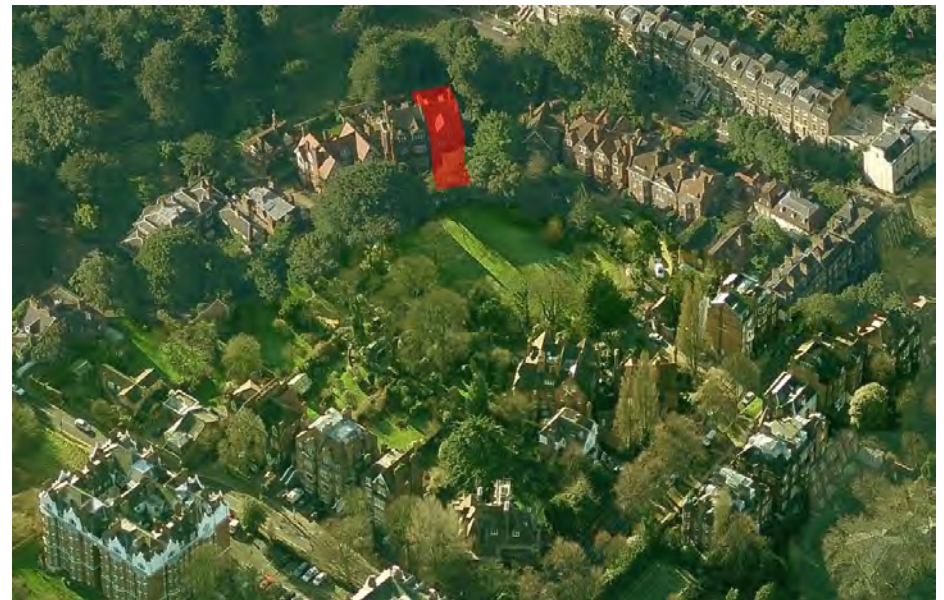
Figure 6: View from the north, showing the front elevation of no.8 Gainsborough Gardens- highlighted red. (Bing maps)
