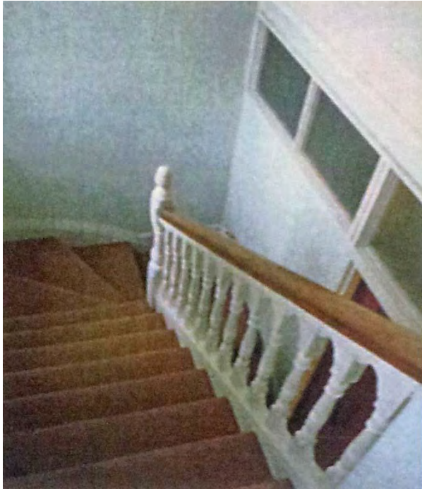
Figure 15: Staircase prior to the removal of the internal partitions (Greenway and Lee Architects – Supporting Planning, Design and Access Statement, 2007)
