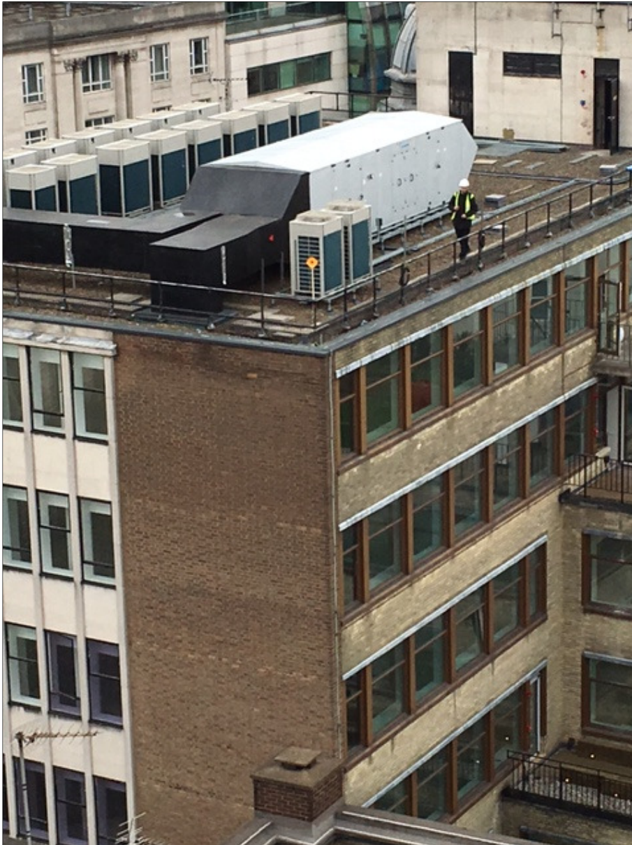
North core as viewed from the neighbouring position
