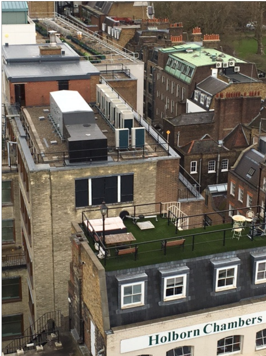
South core as viewed from the neighbouring position
