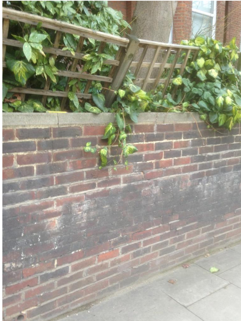
Photo No. 2 to show wall cracking (2) adjacent to Norway maple T2 (trunk visible). Note yellow pencil for scale.
