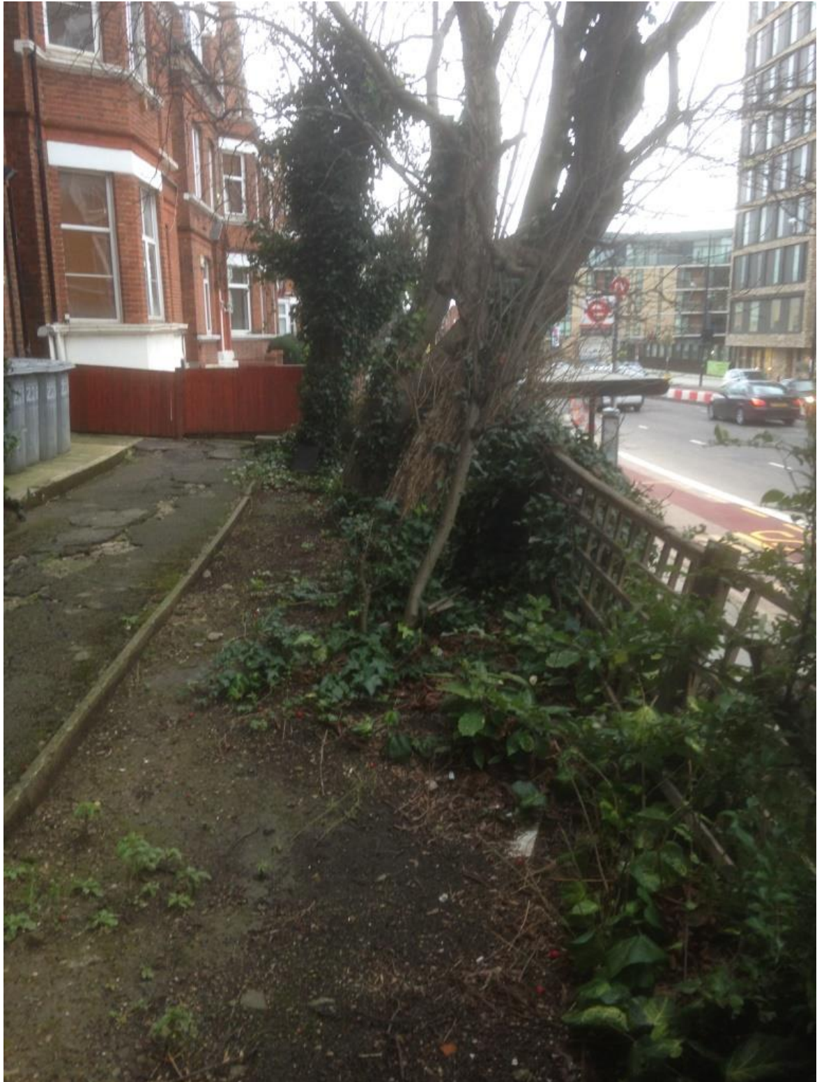
Photo No 3. To show leaning trunks on T3 and T4 (looking south)
