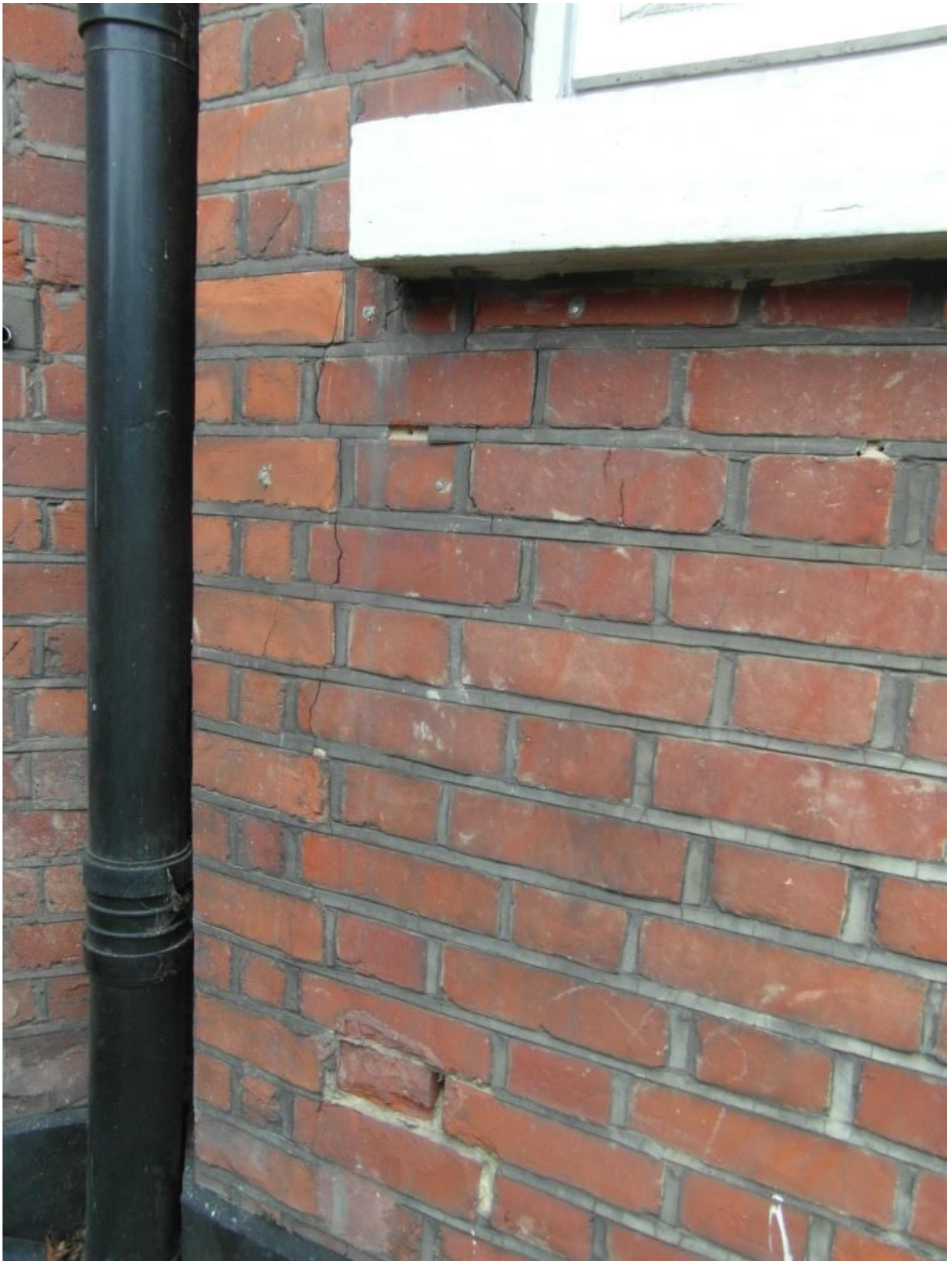
Main Building Bay 1
