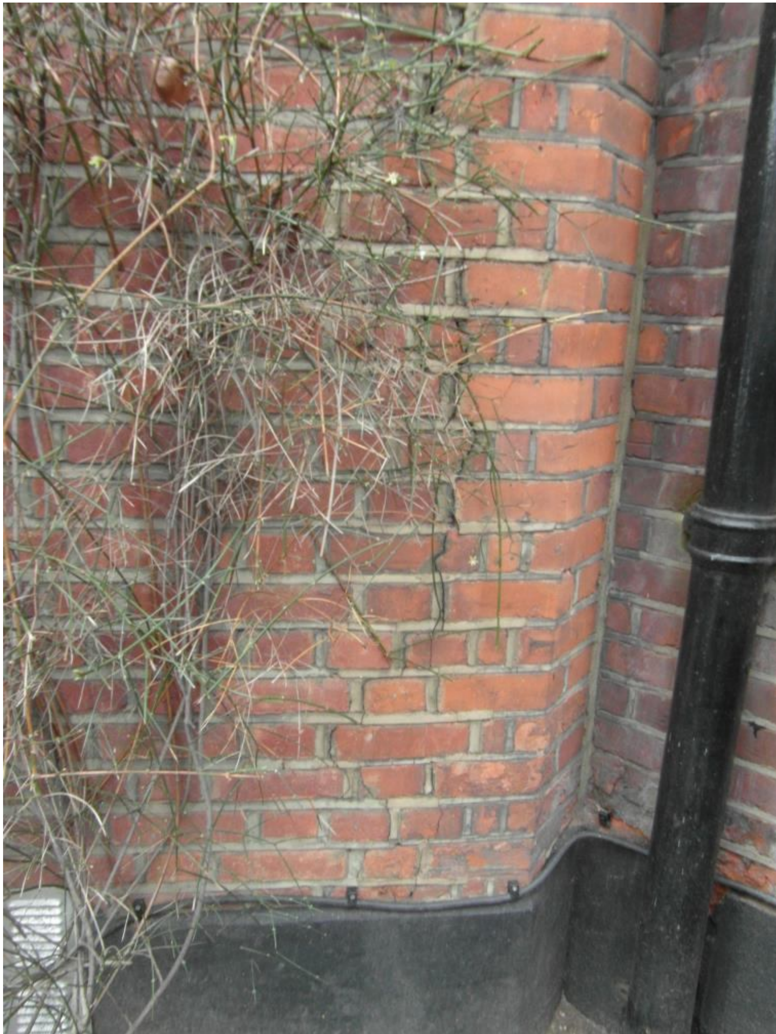
Main Building Bay 2
