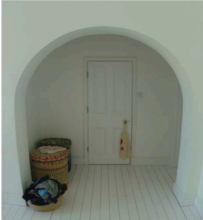
fig.7 Entrance to the main bathroom from first floor landing
