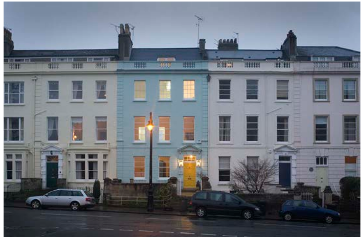
fig.1a Refurbished Grade II listed façade
