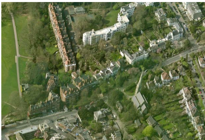
fig.4 Aerial view of south section of Highgate West Hill.
