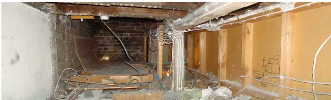
fig.8 Void between original first floor ceiling joists & modern bathroom ceiling
