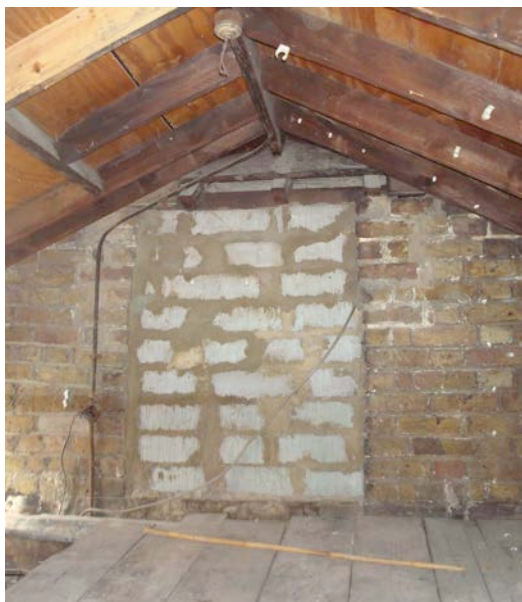
fig.11 Boundary wall to 11a within roof space
