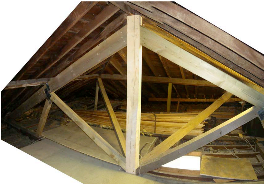
fig.9a Modern timber truss replacement
