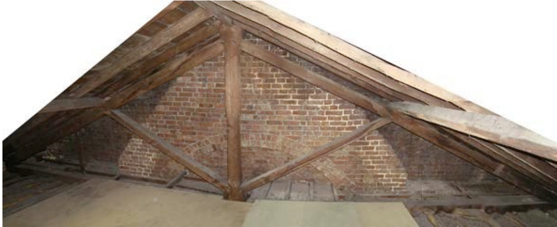
fig.9 Original Kingpost truss adjacent to chimney stack
