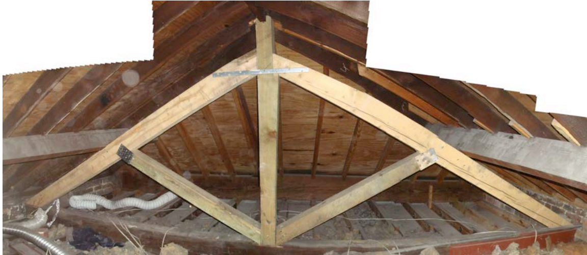
fig.10 Modern timber truss replacement
