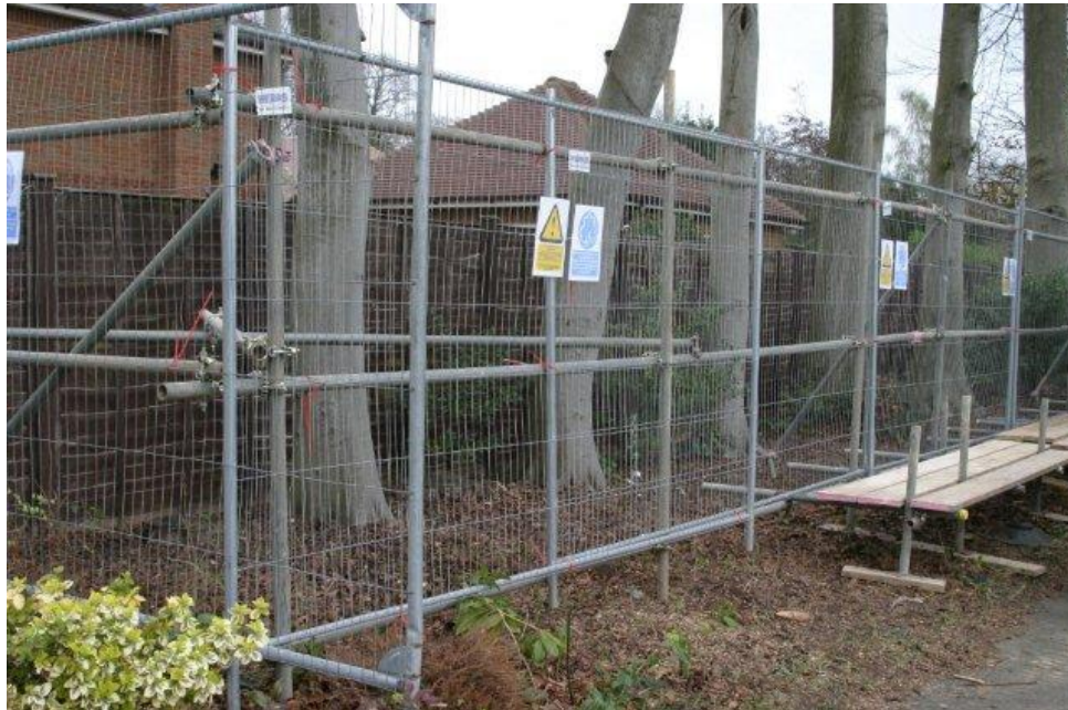
Figure 2: An example of 'floating' ground protection
