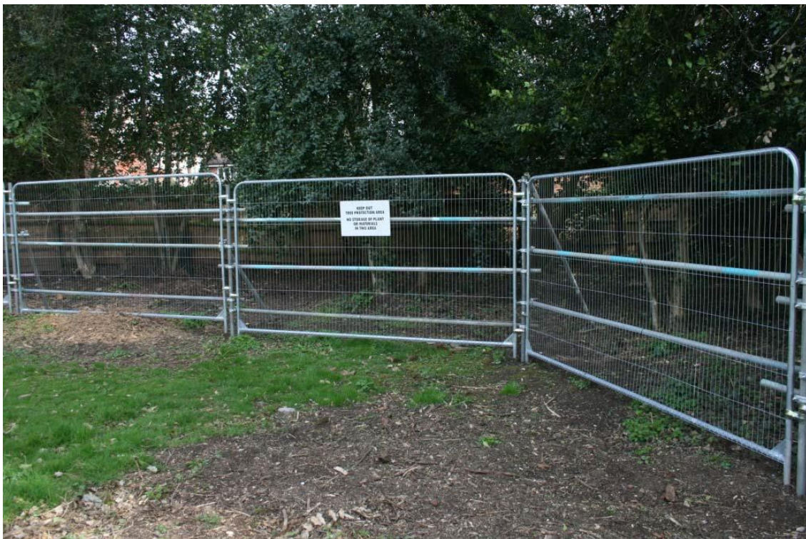
Figure 3: An example of protective fencing erected to the correct specification
