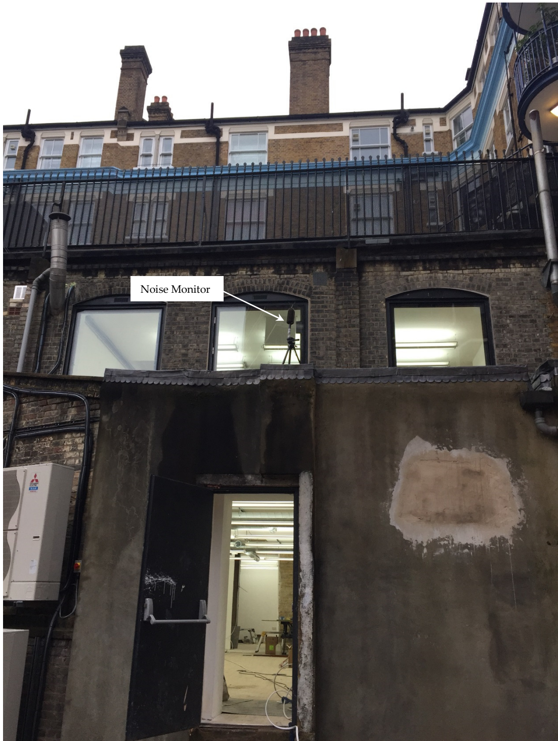
Figure A.4: Noise Monitoring Equipment at rear of 10c Warner Street
