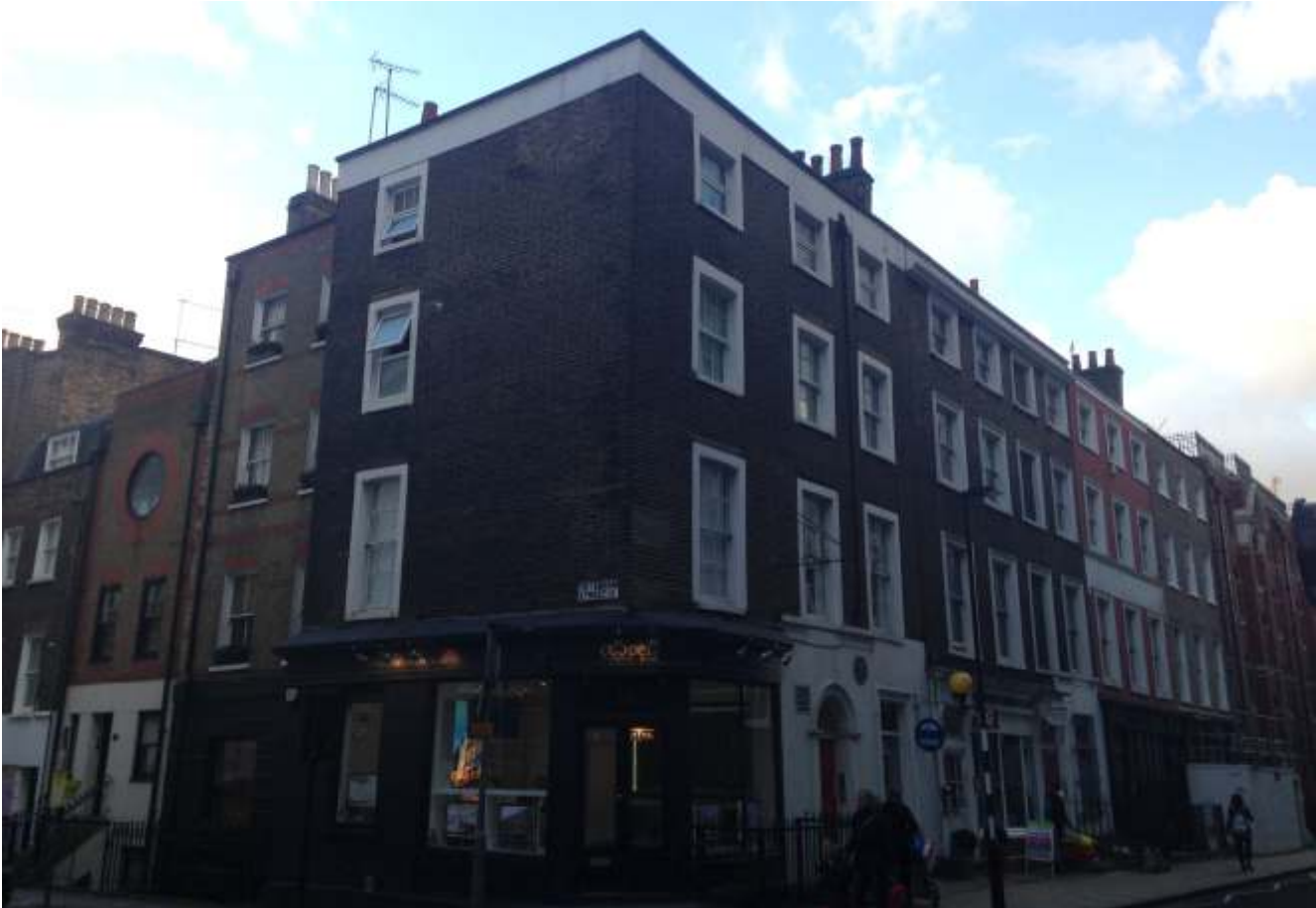
Appendix 1.1: View of front and side elevations of No. 22 Cleveland Street.
