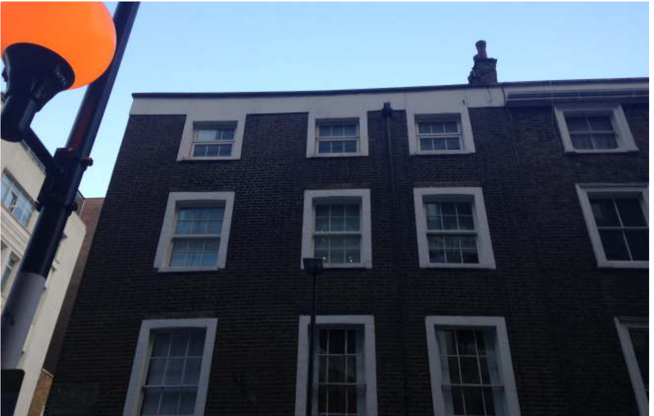
Appendix 1.3: View of front elevation showing new sash windows.
