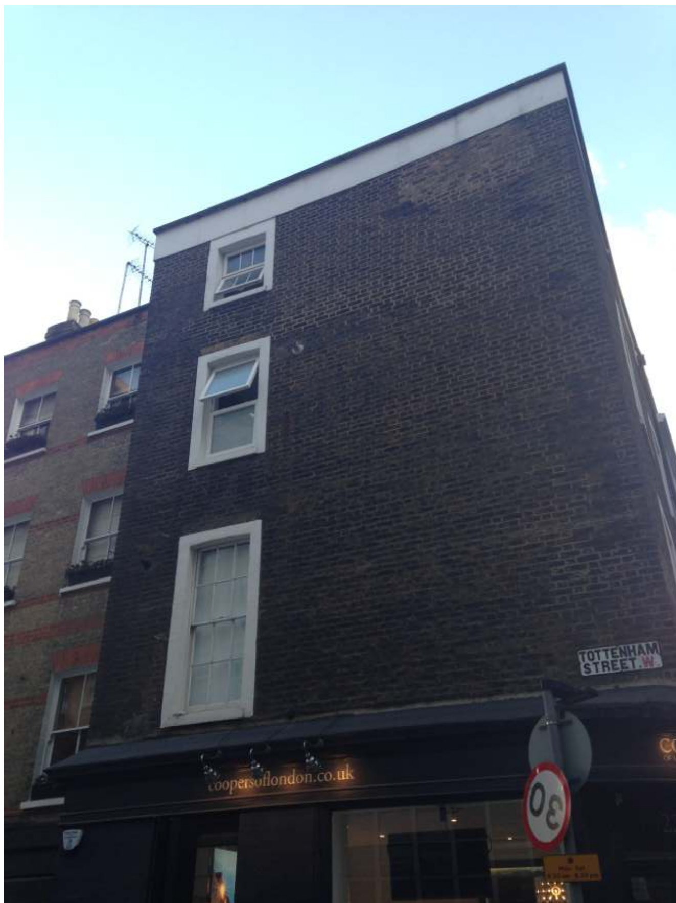
Appendix 1.5: Side view of No. 22 Cleveland Street, showing new window to second floor flat.
