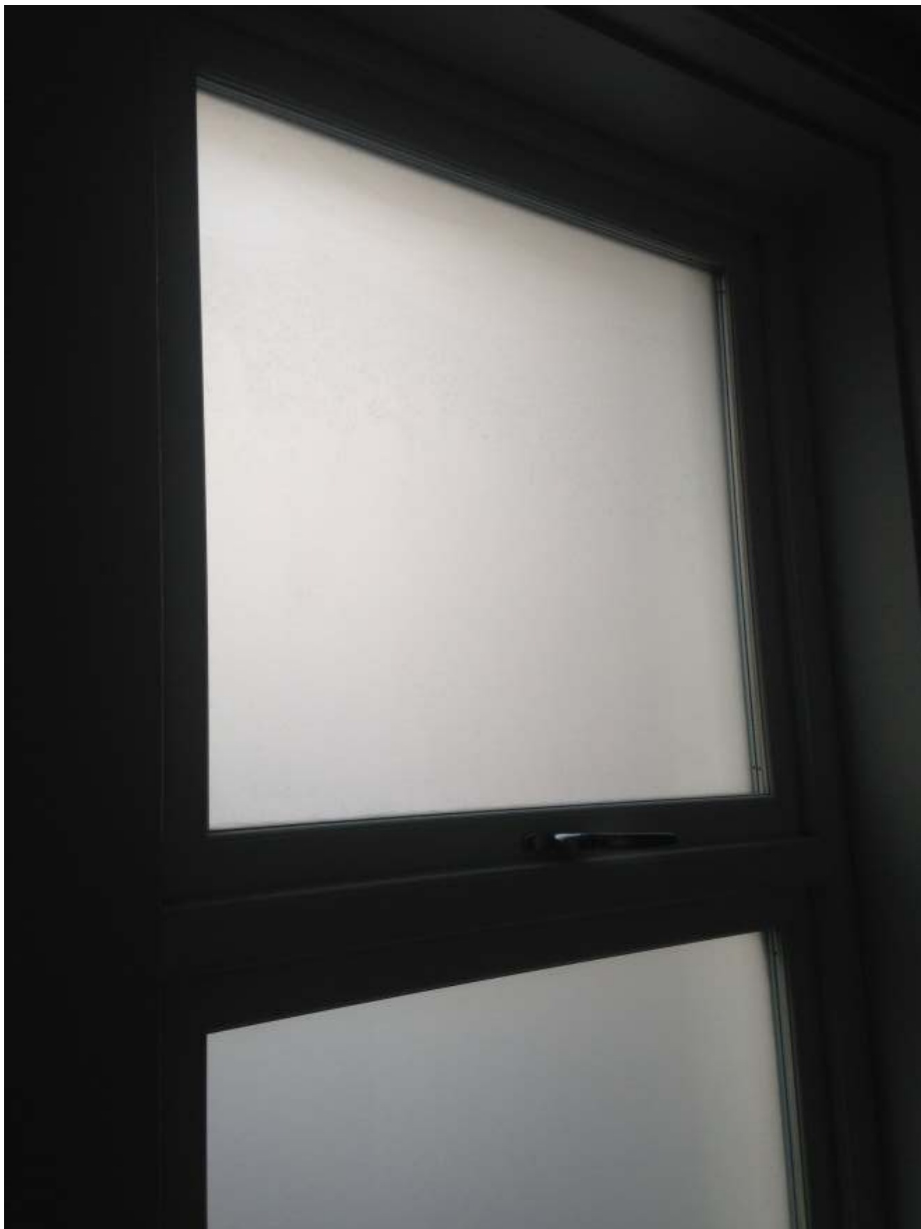
Appendix 1.10: New timber awning window to bathroom of second floor flat.
