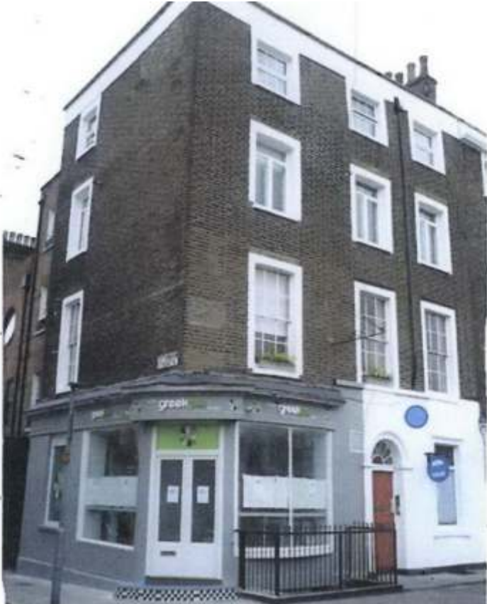
Appendix 1.2: View of front and side elevations of No. 22 Cleveland Street showing previous casement windows to second floor.
