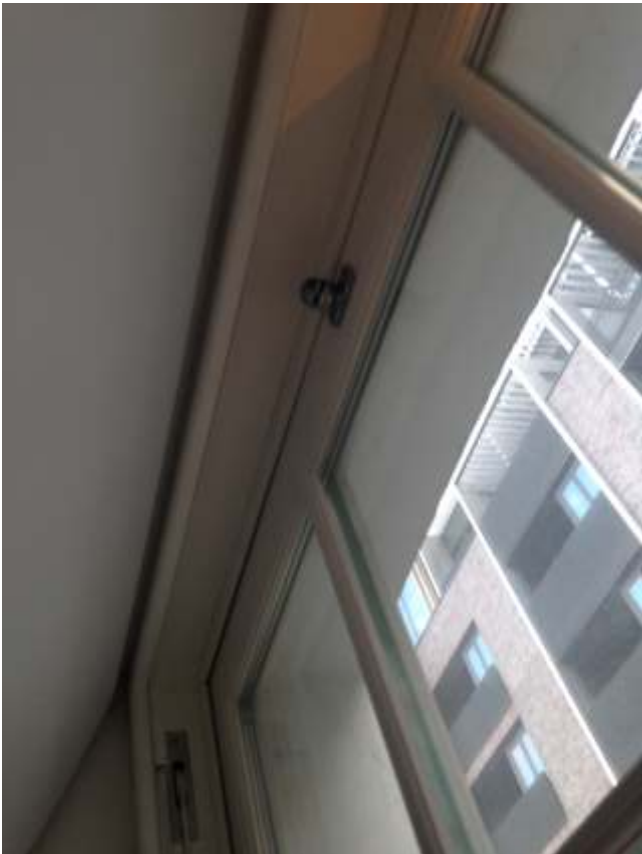
Appendix 1.8: View of top rail and head jamb.
