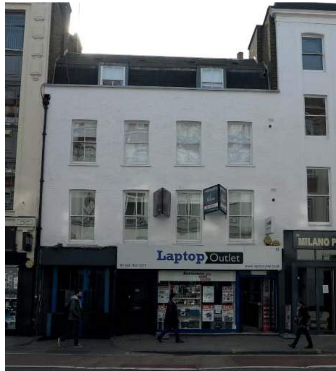
Fig: 2.25 No. 51 TCR - Photo of Existing Elevation
