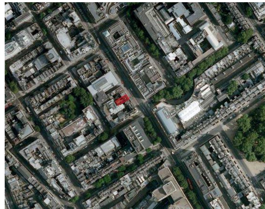
Fig 2.2 Site Aerial Photograph
