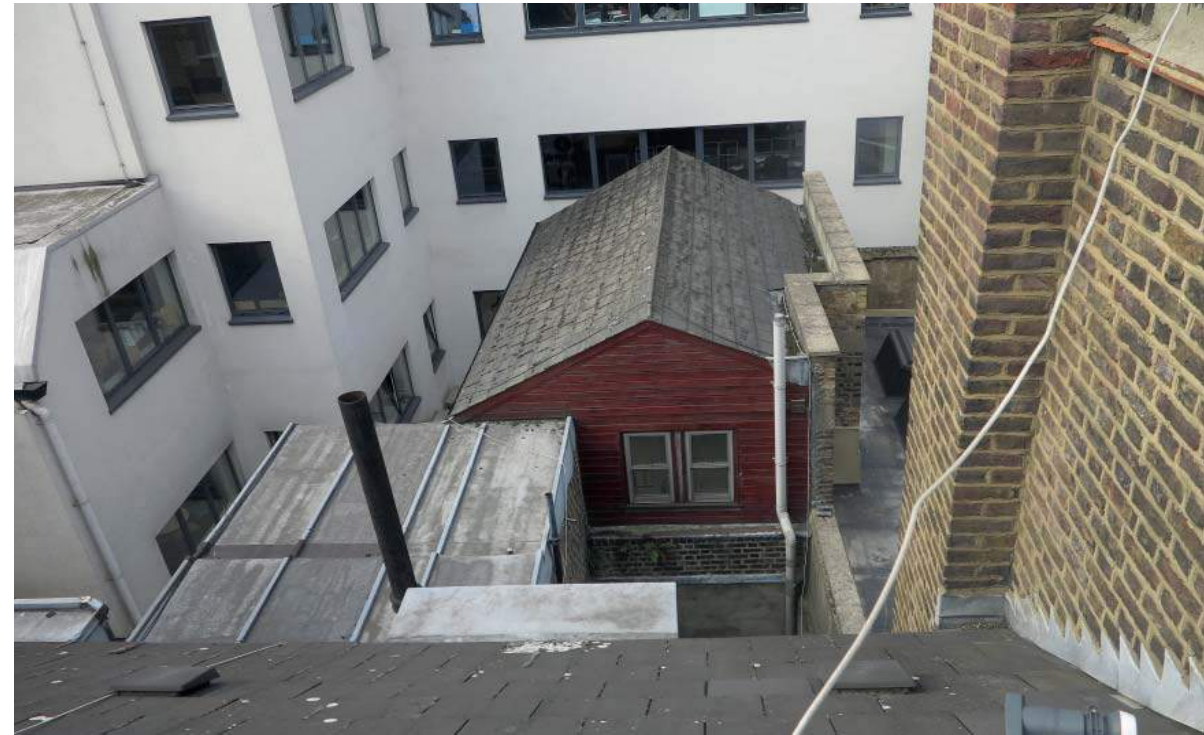
Fig: 2.37 View of rear roof no. 51 - 52 TCR
