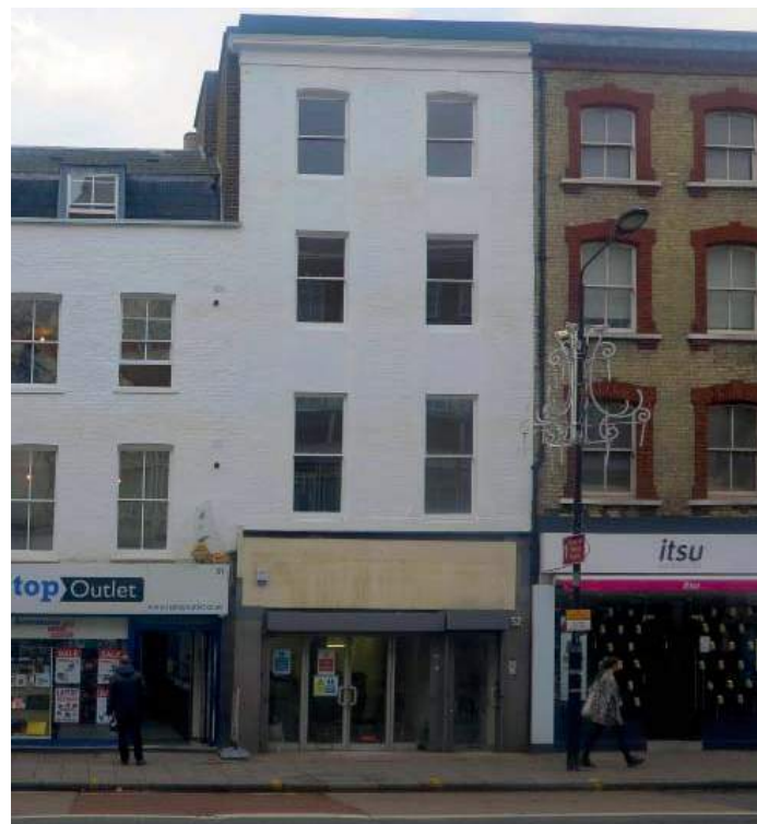
Fig: 2.27 No. 52 TCR - Photo of Existing Elevation
