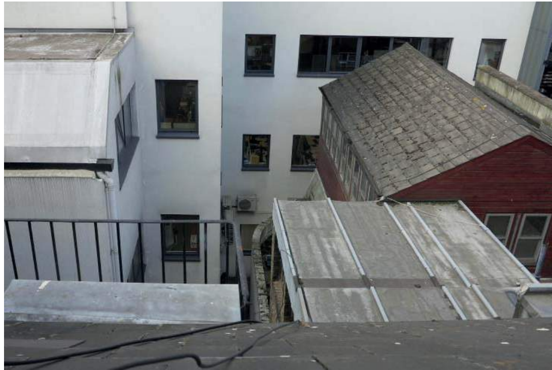
Fig: 2.36 View of rear roof no. 51 TCR
