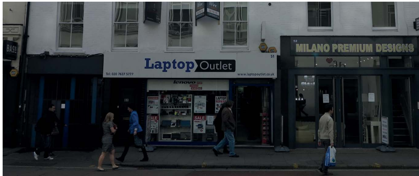
Fig: 2.34 Gated Entrance to no. 50TCR and adjacent shop fronts at no. 51 - 52 TCR
