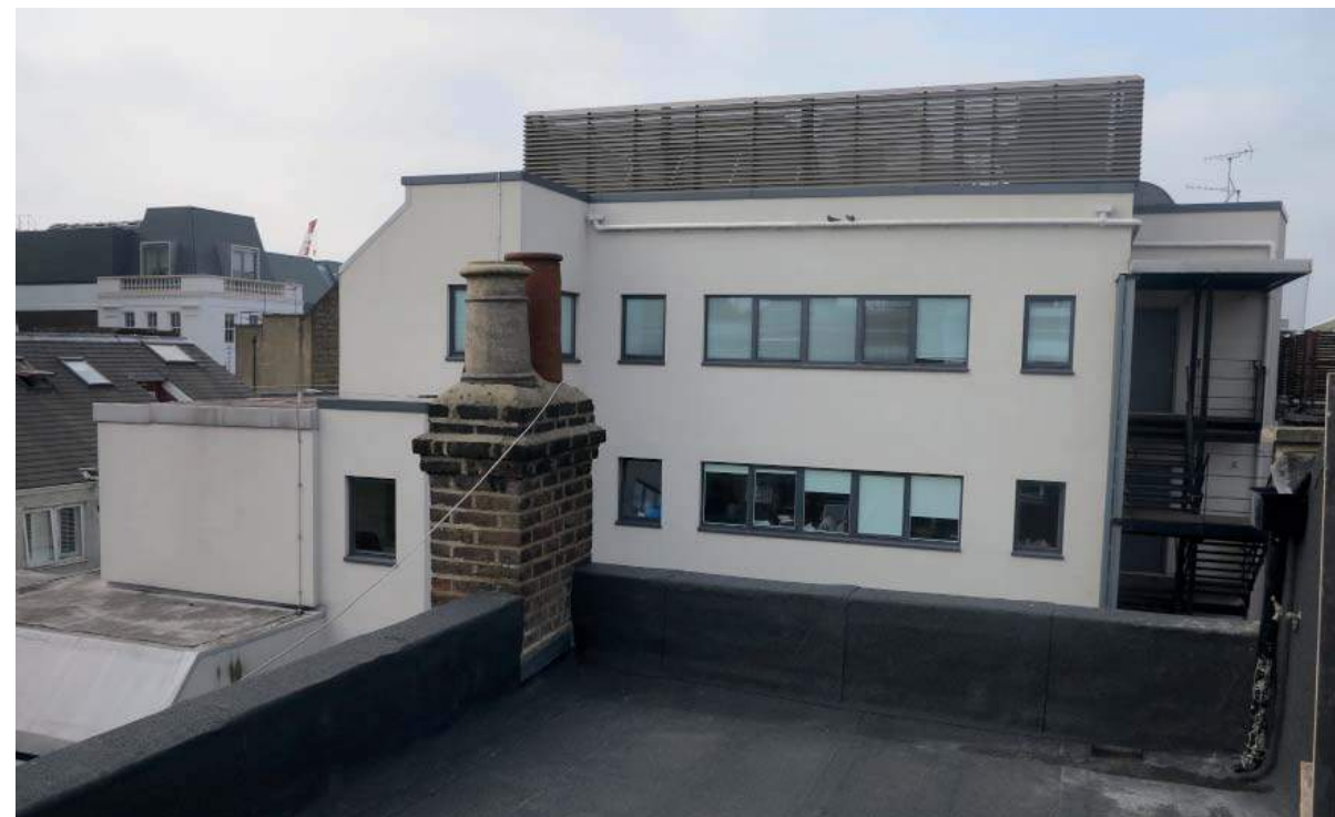
Fig: 2.39 View of rear 6-10 Whitfield St. Photo taken from roof of no. 52 TCR
