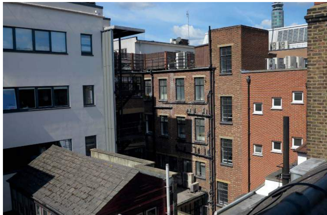
Fig: 2.38 View of rear roof no. 51 TCR, and rear elevations of buildings on Kirkman Place
