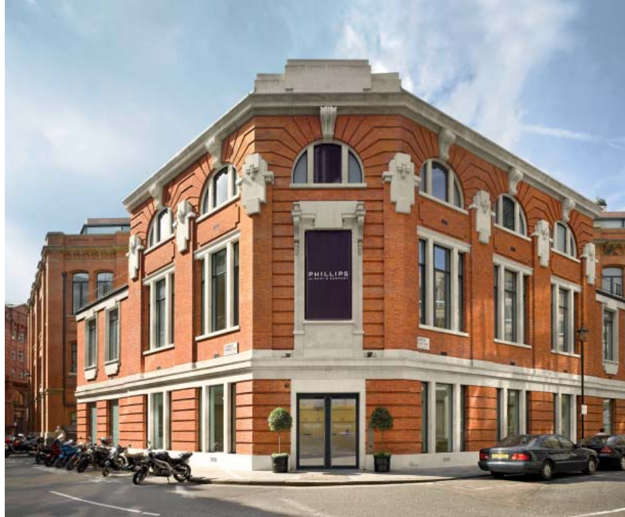
Howick Place - Listed Building Mixed Use Conversion
