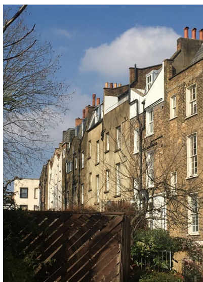
View of the rear elevations
