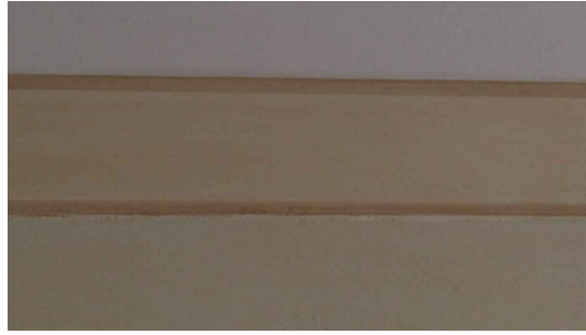
10 EXISTING CORNICE IMAGE SECOND FLOOR EXISTING SECOND FLOOR LANDING
