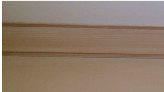
11 EXISTING CORNICE IMAGE THIRD FLOOR TYPICAL THIRD FLOOR
