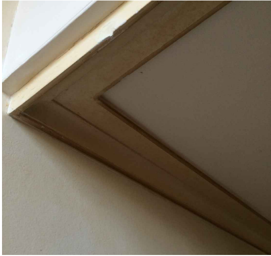
07 EXISTING CORNICE IMAGE FIRST FLOOR EXISTING FIRST FLOOR LANDING
