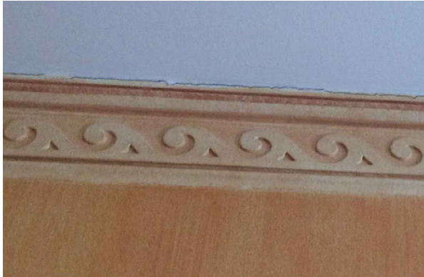
08 EXISTING CORNICE IMAGE SECOND FLOOR EXISTING MASTER CHAMBERS
