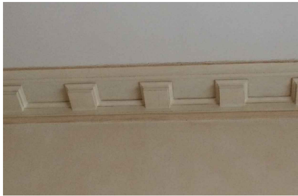
02 EXISTING CORNICE IMAGE GROUND FLOOR EXISTING DINING / DAY ROOM
