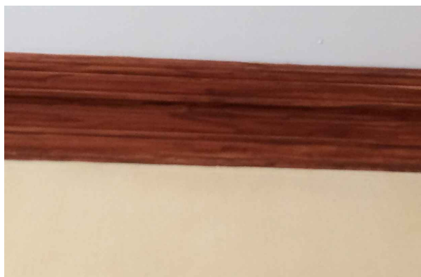
03 EXISTING CORNICE IMAGE GROUND FLOOR EXISTING KITCHEN
