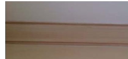
6 | THIRD FLOOR TYPICAL COVING
