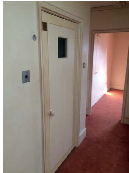
2 | THIRD FLOOR ELEVATOR DOOR
