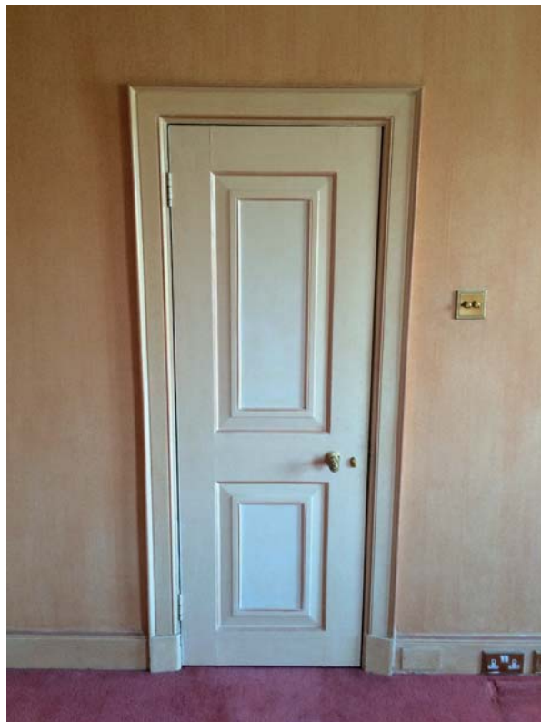
1 | SECOND FLOOR ENSUITE DOOR FROM BEDROOM
