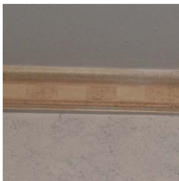
6 | SECOND FLOOR BACK BEDROOM COVING DETAIL
