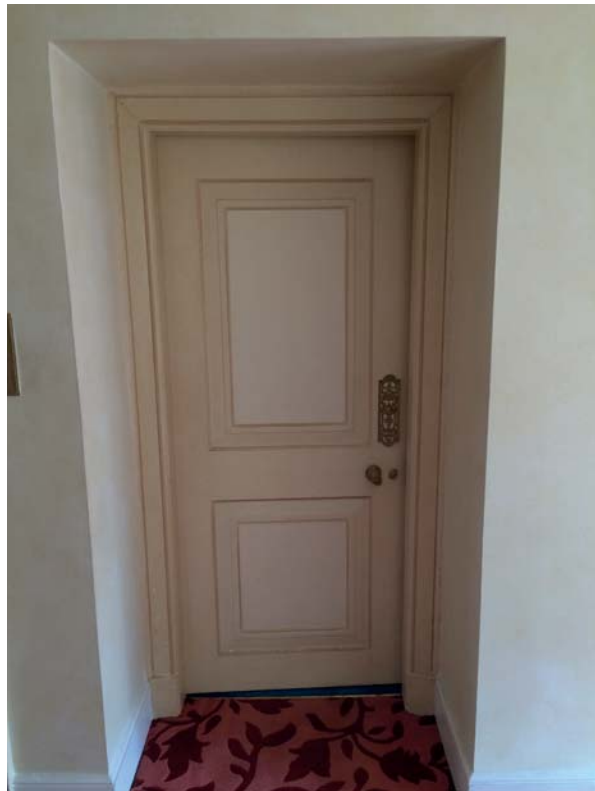
1 | SECOND FLOOR BACK BEDROOM DOOR
