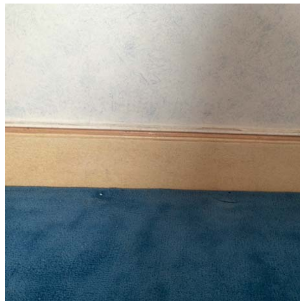
5 | SECOND FLOOR BACK BEDROOM SKIRTING
