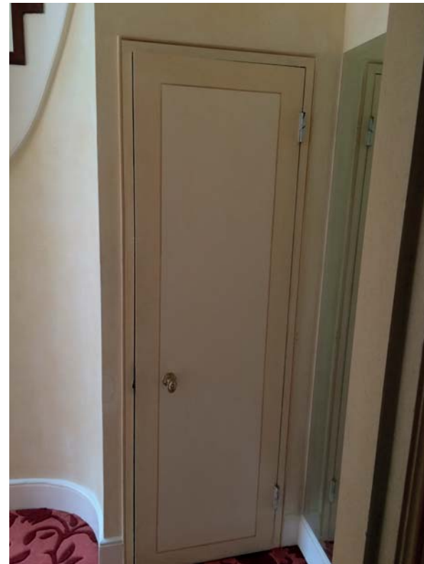
3 | SECOND FLOOR EXISTING BATHROOM DOOR
