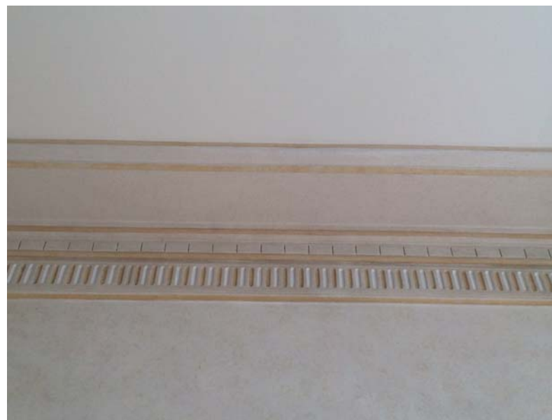
5 | FIRST FLOOR RECEPTION COVING
