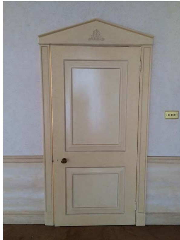
2 | FIRST FLOOR RECEPTION DOOR (VIEW FROM INTERIOR)
