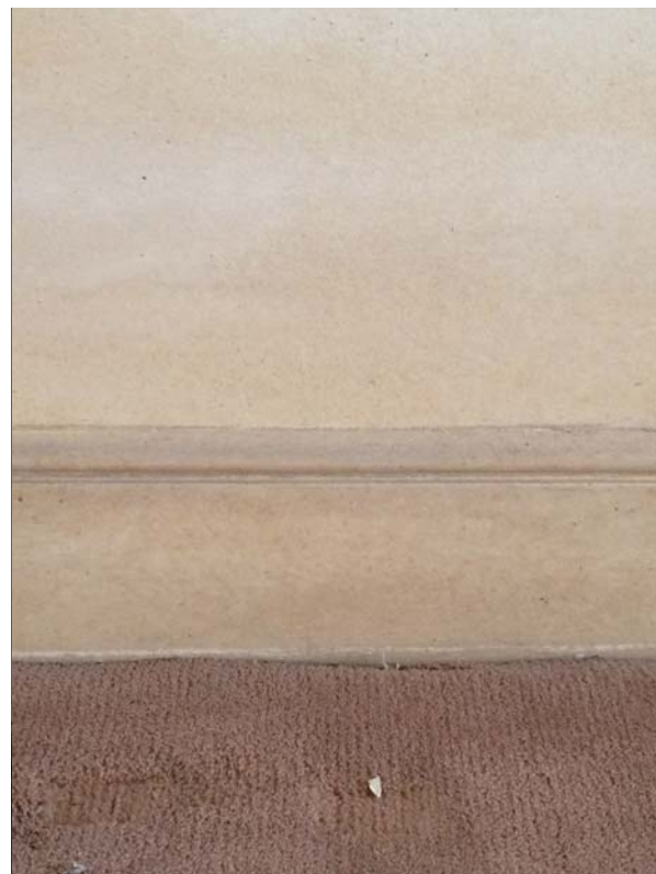
4 | FIRST FLOOR RECEPTION SKIRTING
