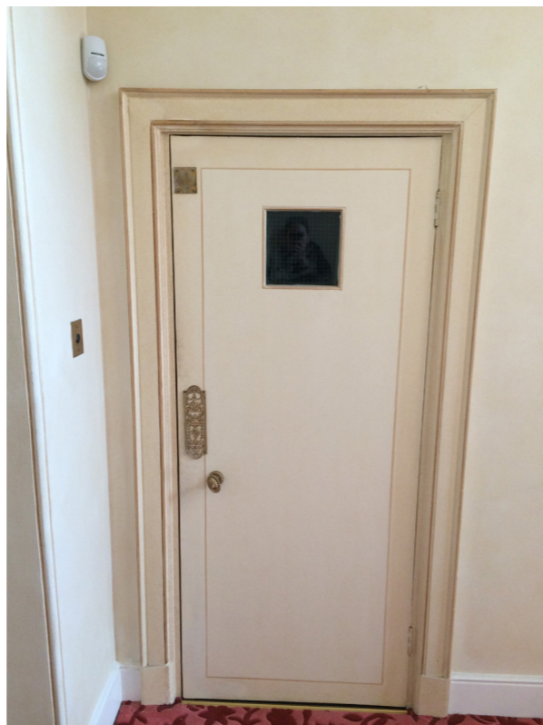
5 | FIRST FLOOR ELEVATOR DOOR
