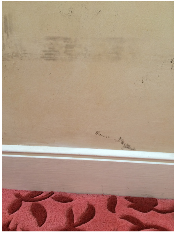
1 | FIRST FLOOR STAIRWELL SKIRTING
