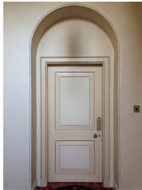
6 | FIRST FLOOR MIAN RECEPTION DOOR FROM STAIRWELL
