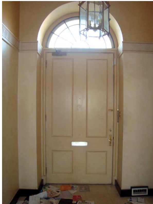
1 | GROUND FLOOR FRONT DOOR IN ENTRY
