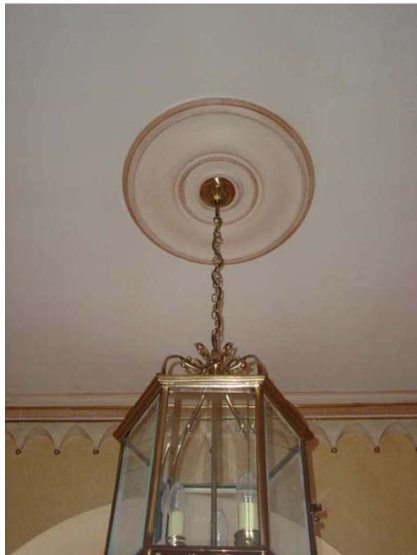
2 | GROUND FLOOR FRONT VESTIBULE CEILING ROSE
