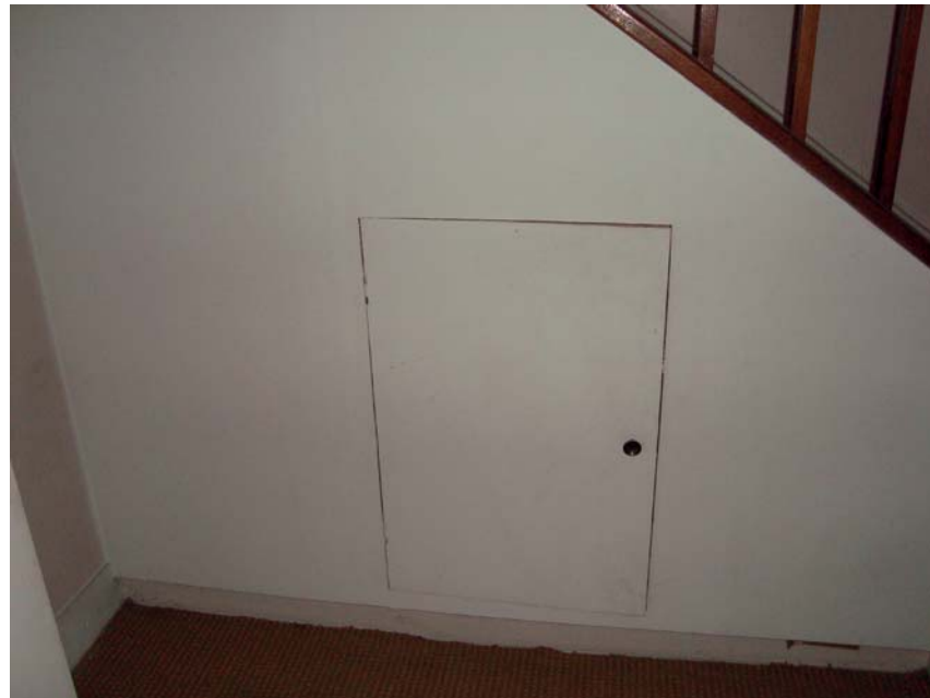
5 | LOWER GROUND FLOOR UNDER STAIR CUPBOARD
