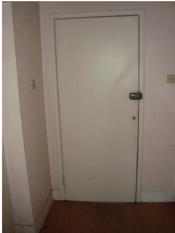
1 | LOWER GROUND FLOOR BACK EXIT DOOR
