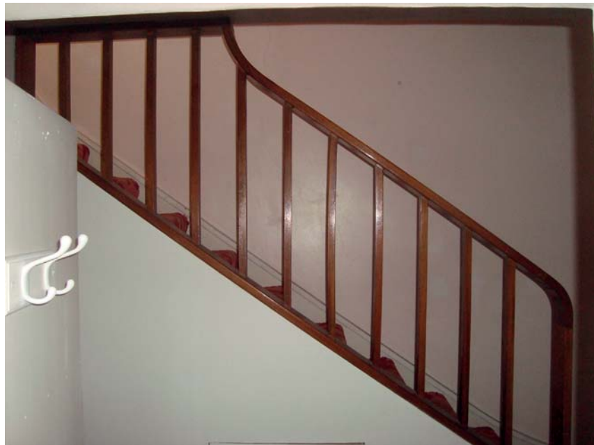
4 | LOWER GROUND FLOOR RAILING OVERVIEW
