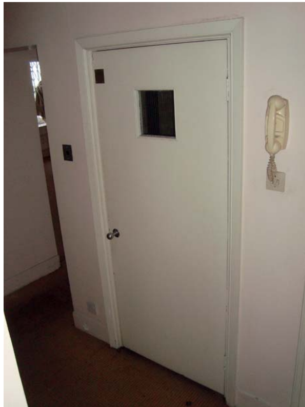
2 | LOWER GROUND FLOOR ELEVATOR DOOR
