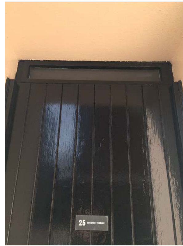
3 | EXTERIOR LW. GR. BACK DOOR DETAIL
