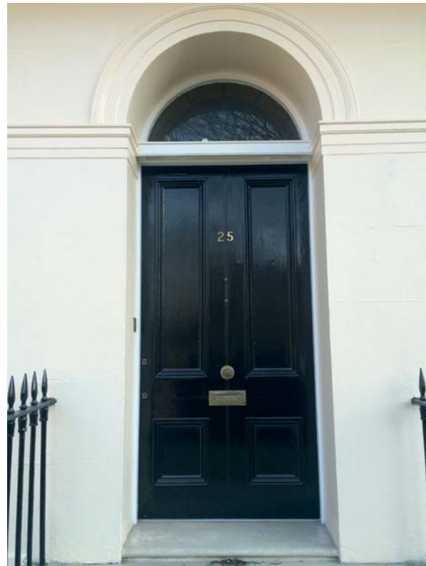
2 | EXTERIOR GR. FL. FRONT DOOR
