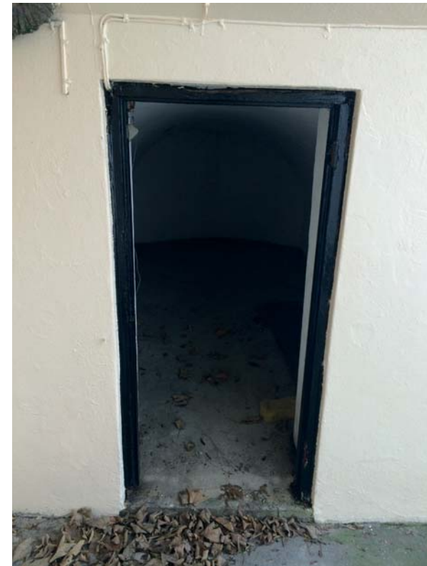
6 | EXTERIOR LEFT VAULT (NO EX. DOOR)
