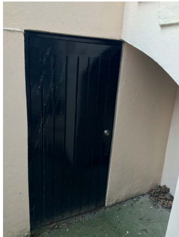
4 | EXTERIOR RIGHT VAULT
