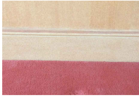
05 EXISTING SKIRTING IMAGE SECOND FLOOR EXISTING MASTER CHAMBERS
