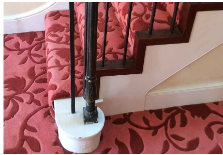
06 EXISTING SKIRTING IMAGE SECOND FLOOR EXISTING STAIR TO THIRD FLOOR
