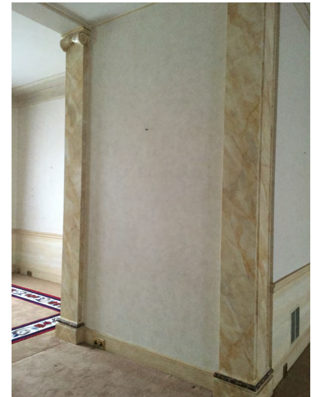
Plate 9: First Floor columns
