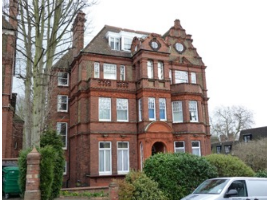
View of front of No. 22 Lyndhurst Gardens (Development flat not visible from this view - forms basement)
