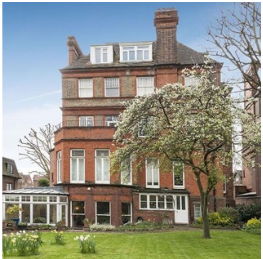
View of rear of No 22 Lyndhurst Gardens showing garden level flat.
