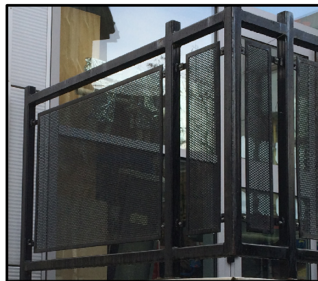
Existing balcony railings to be re-used.
