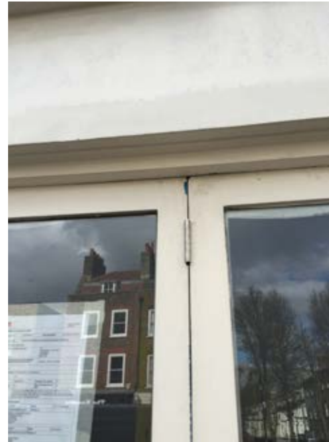
Chipped paint to framework
