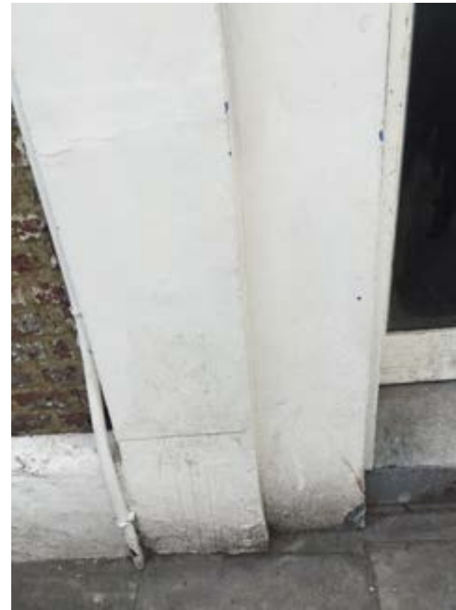
Low level paint chipped at entry point
