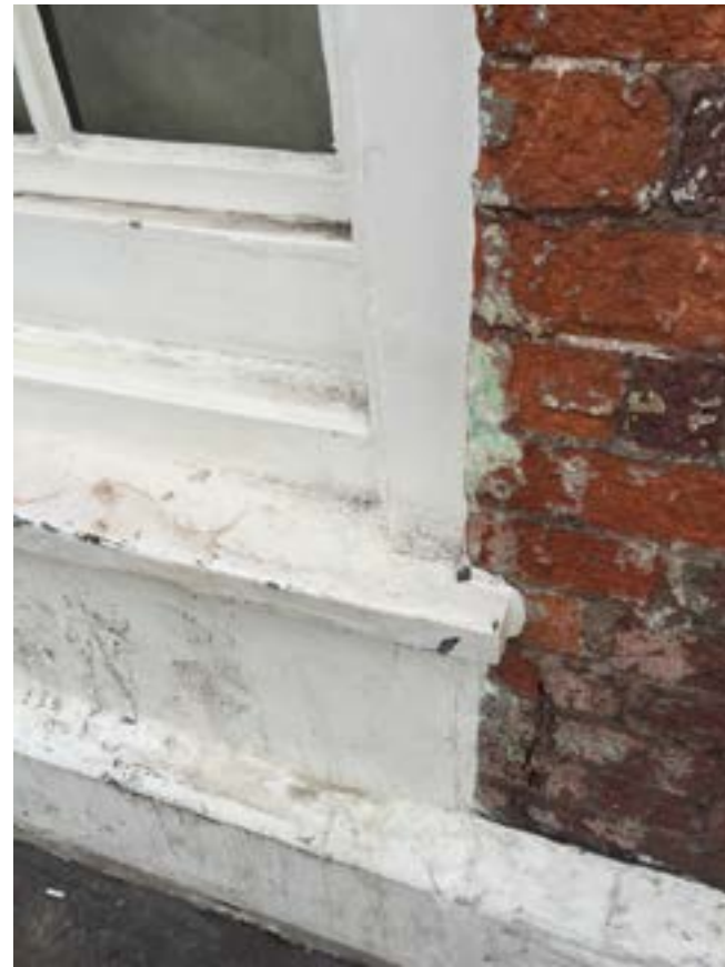
Clean and make good to framework and windows
