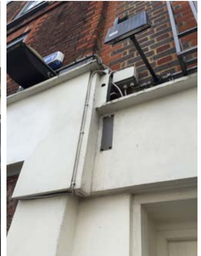
Repair required to patch up old signage locations
