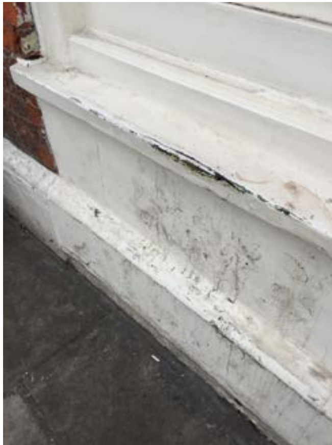
Clean and make good stall riser and sills
