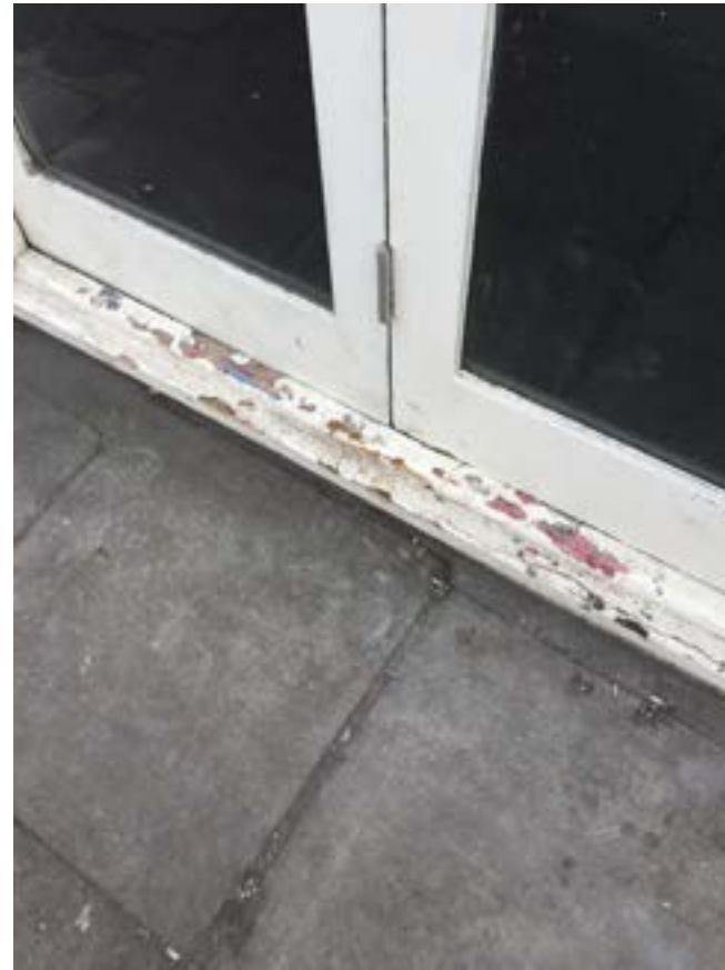
Existing threshold and frame chipped requires weather sealing
