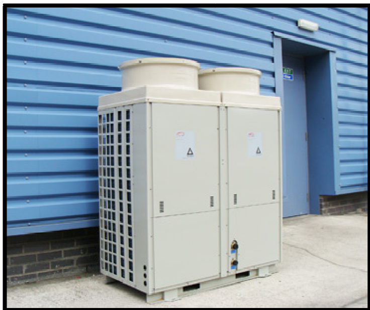
Figure 5 – Air Source Heat Pump Units Example
